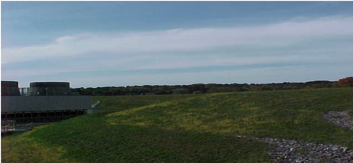
Description: View of Building 71 OPCA plateau (looking west)
