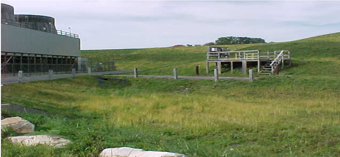
Description: View of Building 71 OPCA and Southern Stormwater Basin (looking north)
