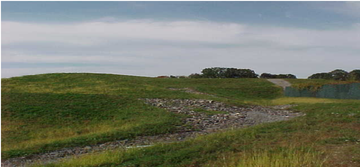
Description: View of Building 71 OPCA (looking north)
