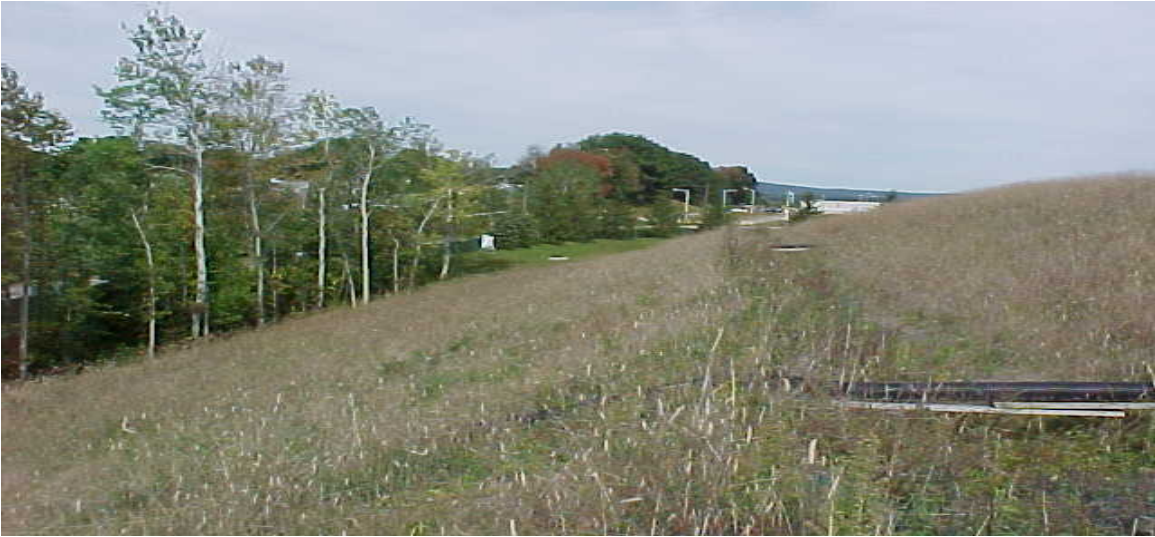
Description: View of Hill 78 OPCA northern sideslope (looking east)
