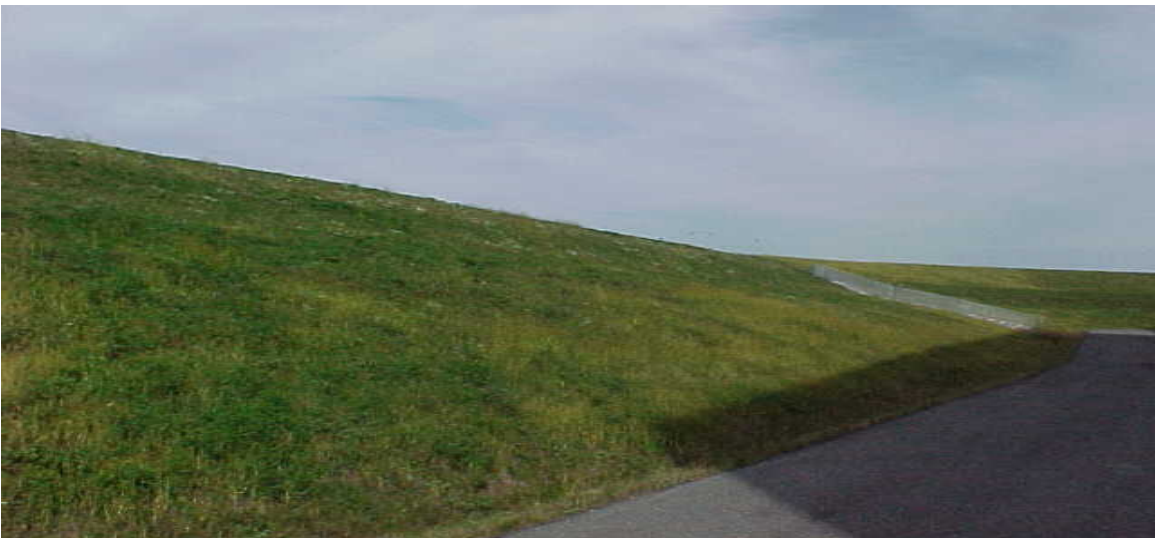
Description: View of Building 71 OPCA southern sideslope (looking east)
