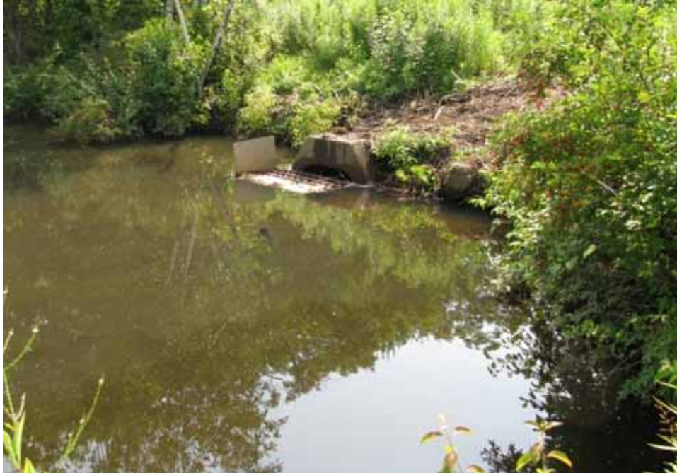
Figure F-11b. Upstream end of culverts beneath the rail spur.
