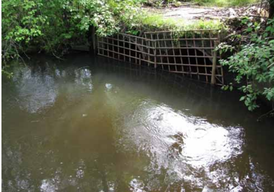
Figure F-11c. Upstream end of culvert located beneath Merrill Road.
