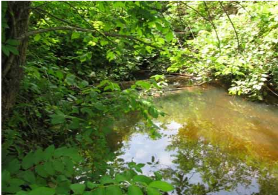
Figure F-11e. Upstream end of railroad culvert.
