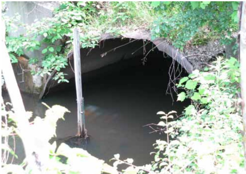
Figure F-11d. Downstream end of underground culvert.
