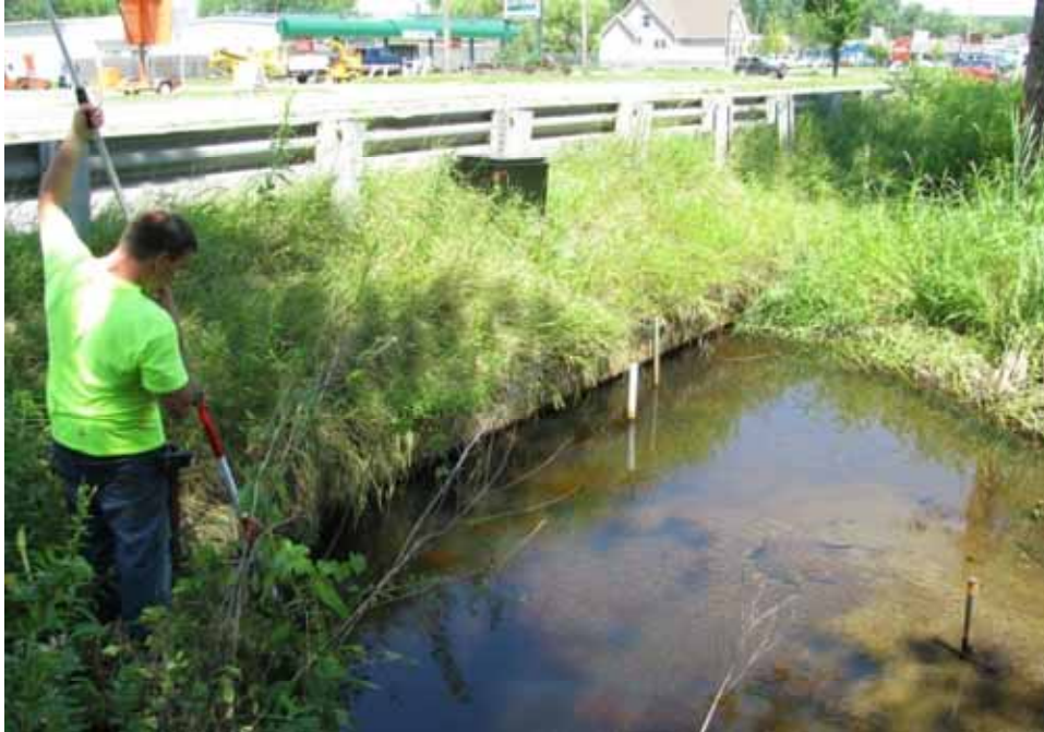
Figure F-11a. Downstream end of culvert located beneath Dalton Avenue.
