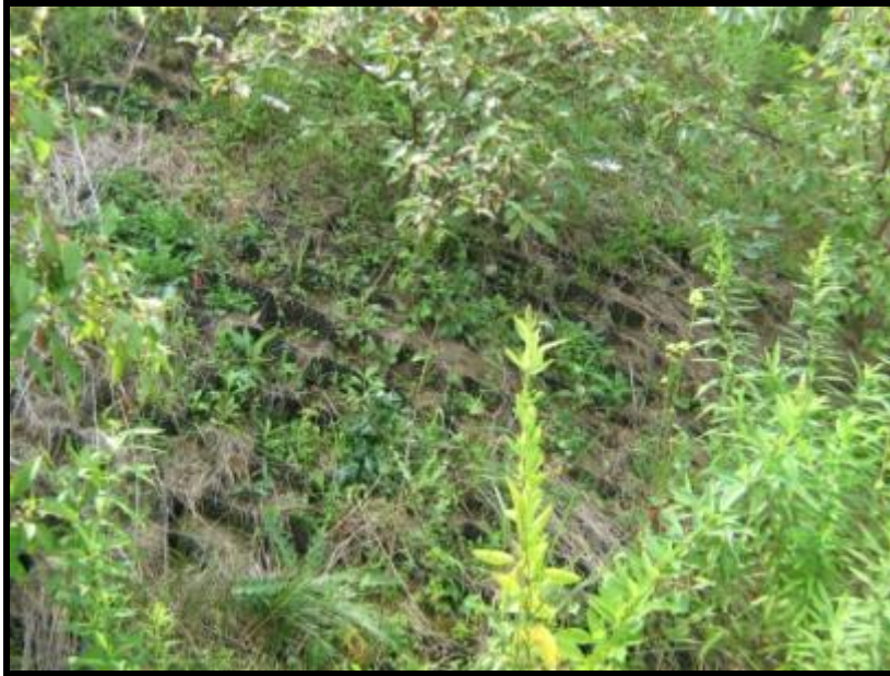
Photograph 7: Area 3A: Exposed Geoweb South on Parcel I8-23-6
