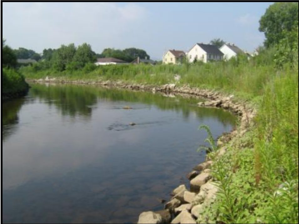
Photograph 1: Wing Wall Deflector and Boulder Cluster
