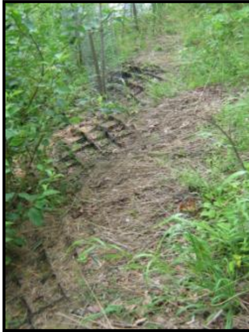
Photograph 8: Area 3: Exposed Geoweb South of Pomeroy Avenue Bridge
