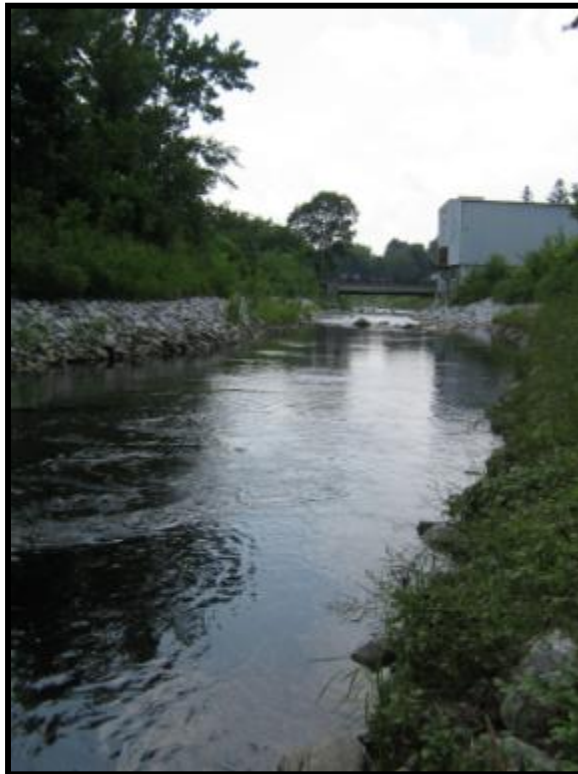
Photograph 10: Pool-Riffle Sequence and Boulder Weir
