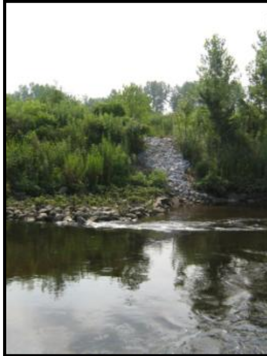
Photograph 3: Riprap Swale and Wing Wall Deflector
