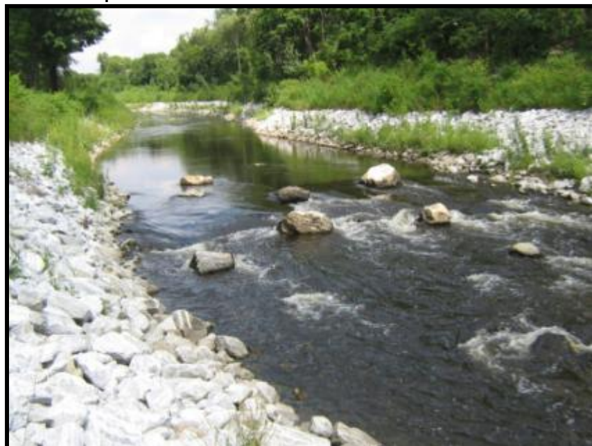
Photograph 10: Pool-Riffle Sequence and Boulder Weir
