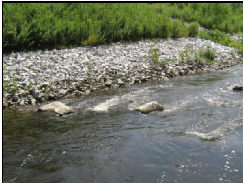
Photograph 8: Pool-Riffle Sequence
