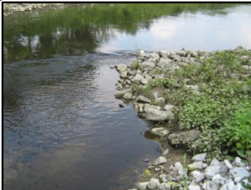
Photograph 4: Wing Wall and Gravel Bar
