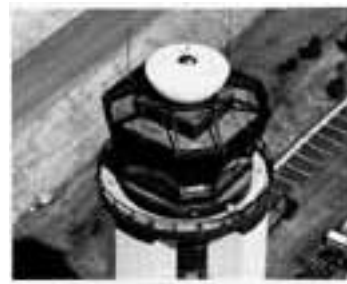
ASDE provides radar surveillance of aircraft and airport service vehicles at high activity airports.
