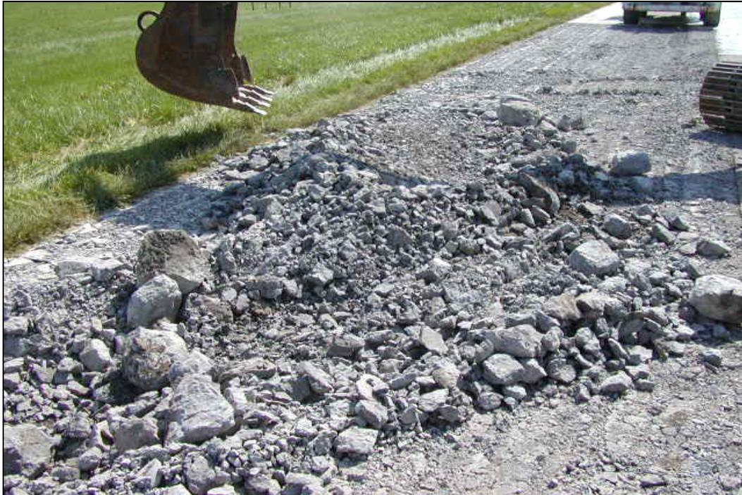
**Figure 5. Inspection Test Pit**
