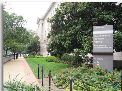
Bioretention cell in front of EPA Headquarters West Building on Constitution Avenue.
