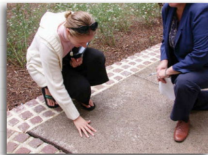
Porous pavement at Ariel Rios South Courtyard.
