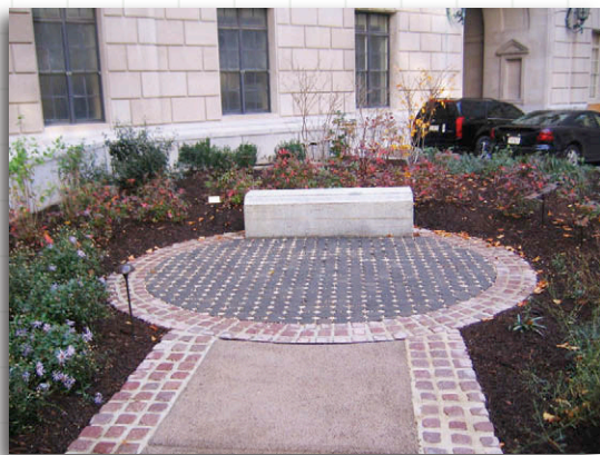
Recycled granite curb used as a bench at the Ariel Rios South Courtyard; permeable pavers used next to bench and permeable concrete used on pathway.
