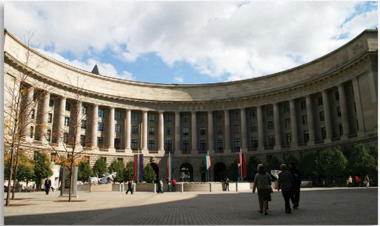
EPA is demonstrating several LID techniques at its Washington, DC Headquarters.
