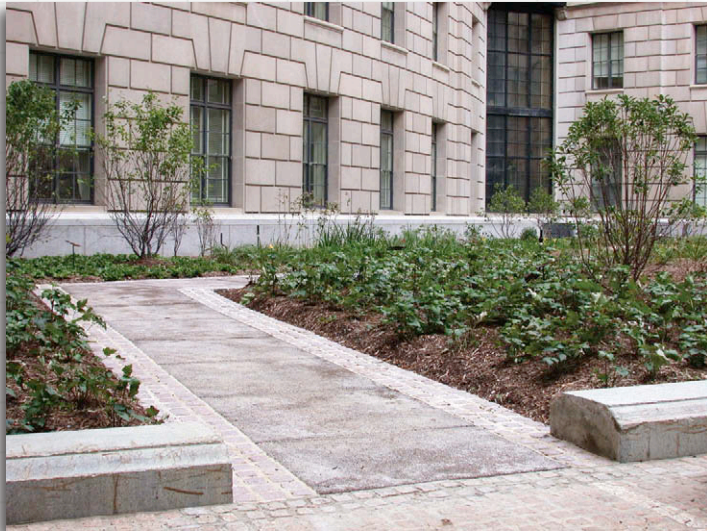
Porous concrete walkway and rain garden at Ariel Rios South Courtyard.
