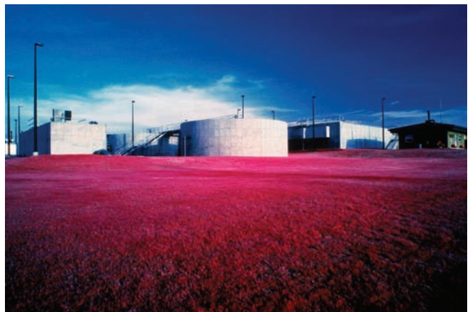
The 2007 Budget provides financial incentives for States to implement permitting fees for municipal and industrial dischargers, such as this wastewater treatment plant. This will result in increased resources for water quality activities across the United States.
