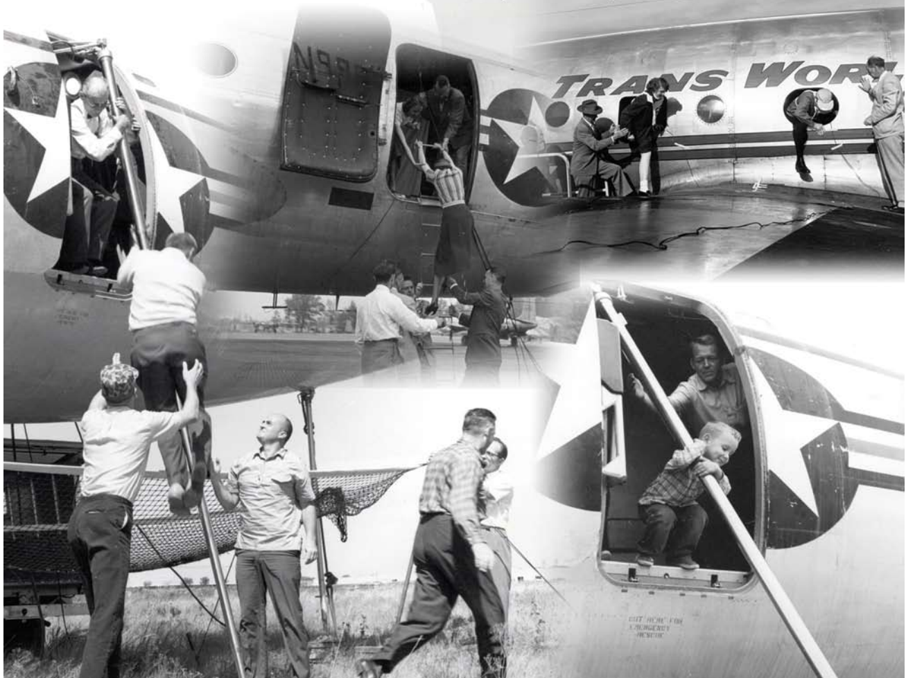
The Way It Was. Into the 1960s, prior to tricycle landing gears and the resulting higher aircraft profiles, emergency escape procedures were rudimentary. Some airlines used ropes and one carrier used a Jacob's ladder. The "telescope" pole (like a fireman's pole, but collapsible for storage) was another approach initially explored. The first escape slides were sheet-like and had to be held by those on the ground.
