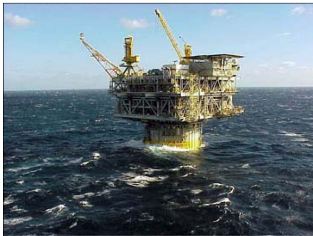
The Deep Draft Caisson Vessel built by Exxon Mobile Corporation is one of the newest offshore drilling and production platforms that are a piece of the critical part of the U.S. oil supply from the Gulf of Mexico. Photo courtesy USCG.
