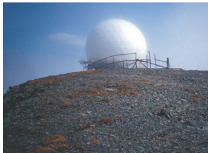
The radar dome at the Cape Newenham LRRS. Woodward Clyde Consultants.
