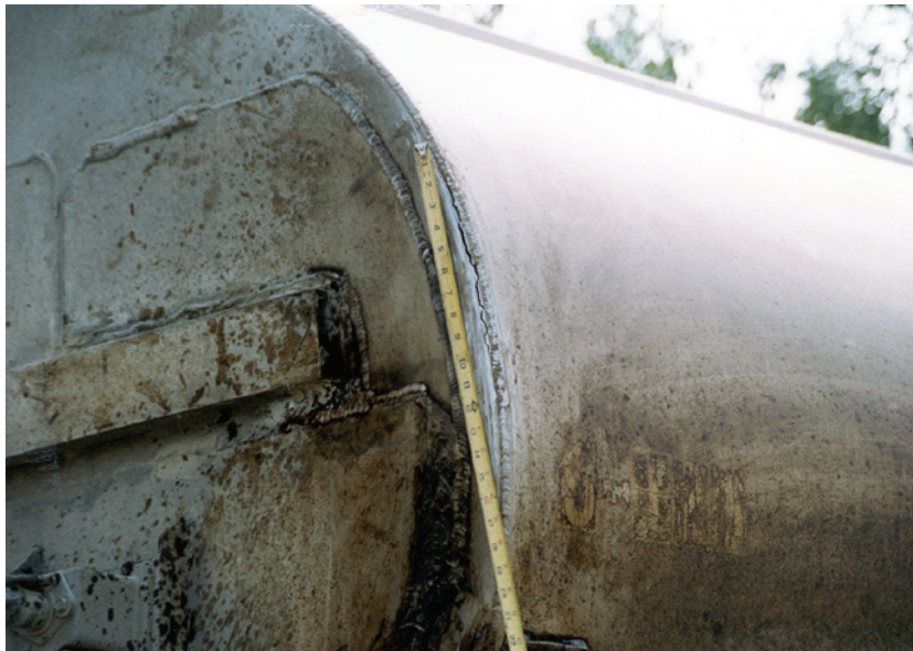
A 14-inch break in the forward bulkhead of this fully loaded tanker resulted in spilled crude oil along Marathon Road within the Beaver Creek Field. USFWS Photo by James E. Frates.
