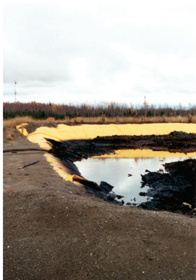
A closer look at one section of the Swanson River Field solid waste facility. USFWS Photo by Tiffany A. S. Parson.
