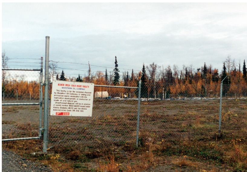
Solid waste facility at Beaver Creek Field. USFWS Photo by Tiffany A. S. Parson.
