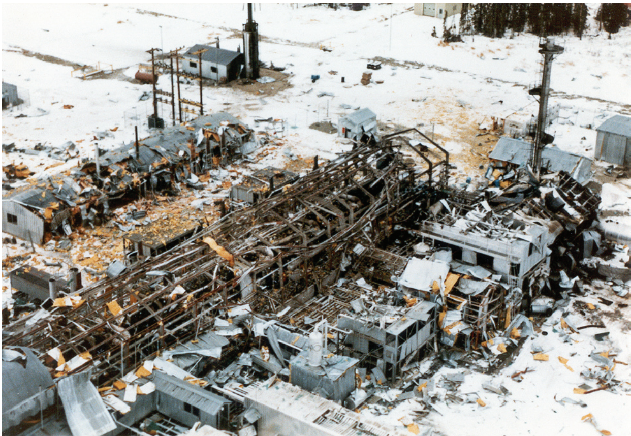
Compressor plant explosion at Swanson River Field on January 26, 1972. The compressor facility (still in operation) provided high-pressure gas for reinjection into oil producing formations, forcing crude to the surface. USFWS Photo by Richard A. Richey.
