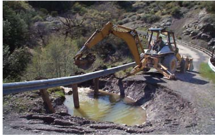
Cooperative road work agreements have increased.
