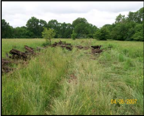
Photo 9: Removal of Railroad Ties
