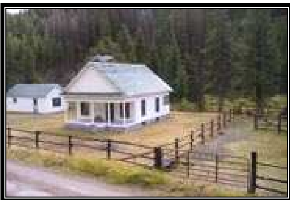
Maintenance at Yellowjacket Rental
