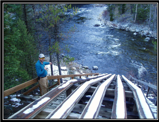
Boundary Creek Ramp Repairs
