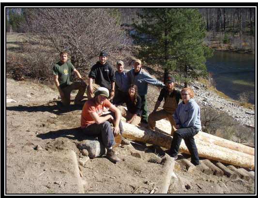
Indian Creek Ramp Repairs
