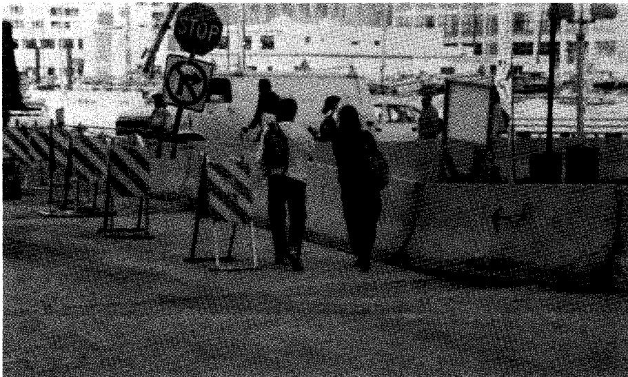
Figure 25. Barrier used to protect pedestrians (Note: Stripes on the barricades are incorrectly oriented in relationship to vehicular traffic).
