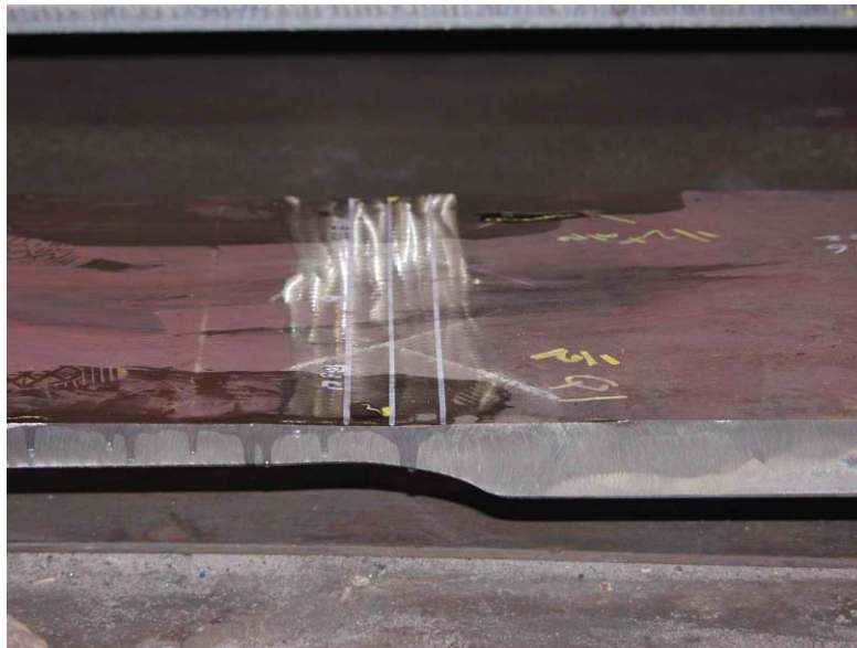
Figure 84. Field specimen G5G-TF1-TopF: Side view of joint.
