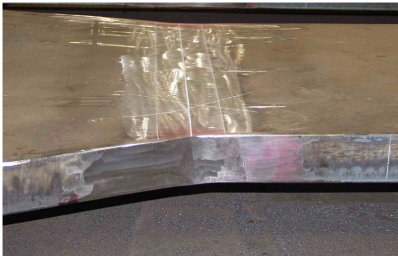
Figure 109. Field specimen FG36K-TF2-TopF-FCM: Side view of joint.
