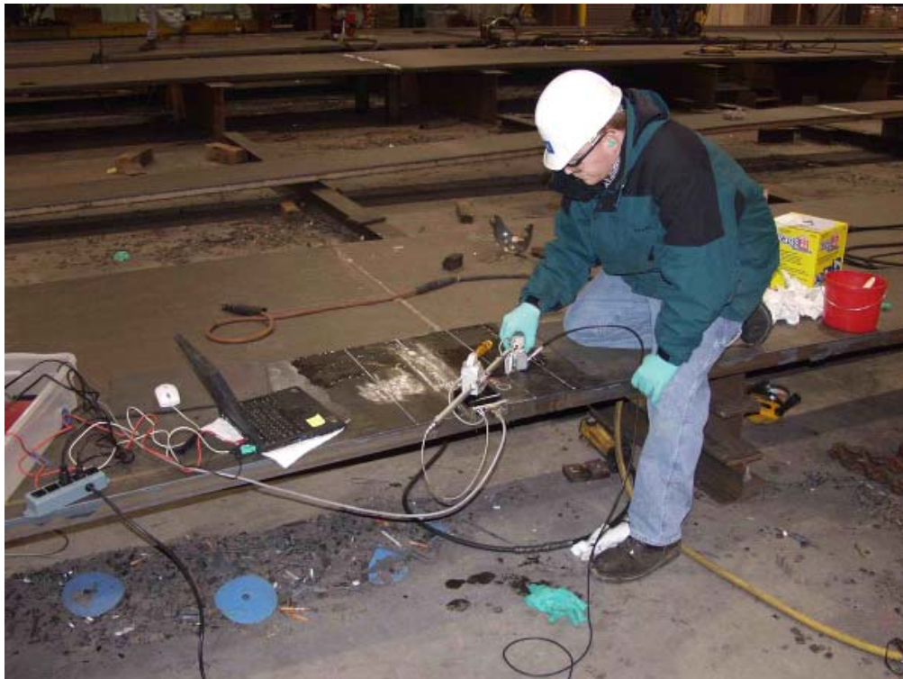
Figure 32. AUT field testing: Stupp Bridge Company.
