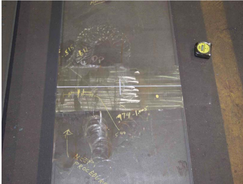
Figure 131. Field specimen FG1A-TF2-BottF-FCM: Top view of joint.
