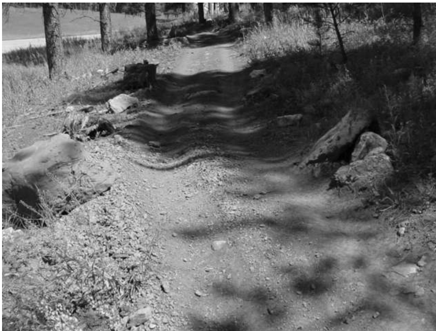
Figure 7. A motorized section of the Centennial Trail less than one year after it underwent an expensive reconstruction
