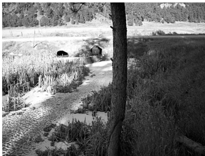
Figure 14. Example of filling across a floodplain creating an effective dike or dam that affects flood flows
