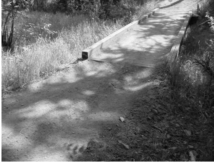
Figure 8. Bridge crossing on motorized section of Centennial Trail
