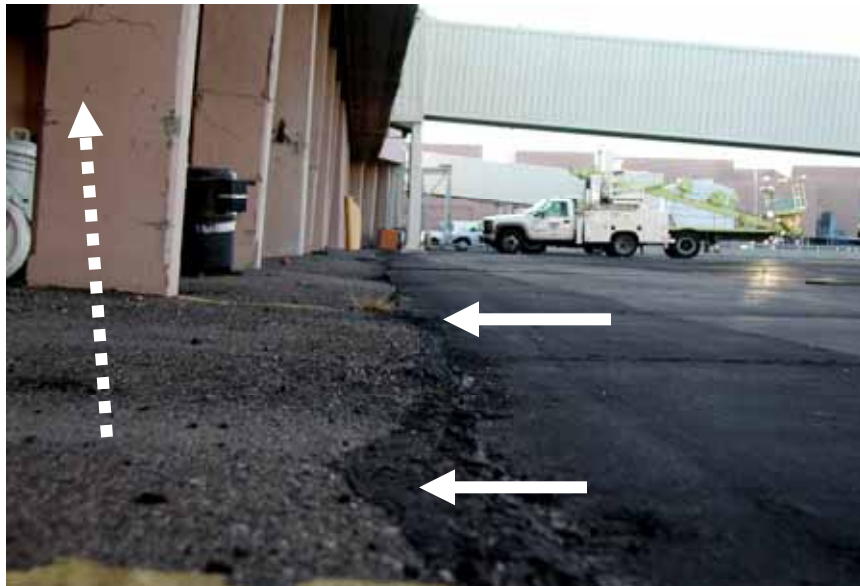
Figure 2-12. Heaving (→) of an asphalt shoulder due to movement of adjoining concrete slab affected by ASR. Movement has been so severe that it has distorted the concrete columns (→) of a neighboring building.
