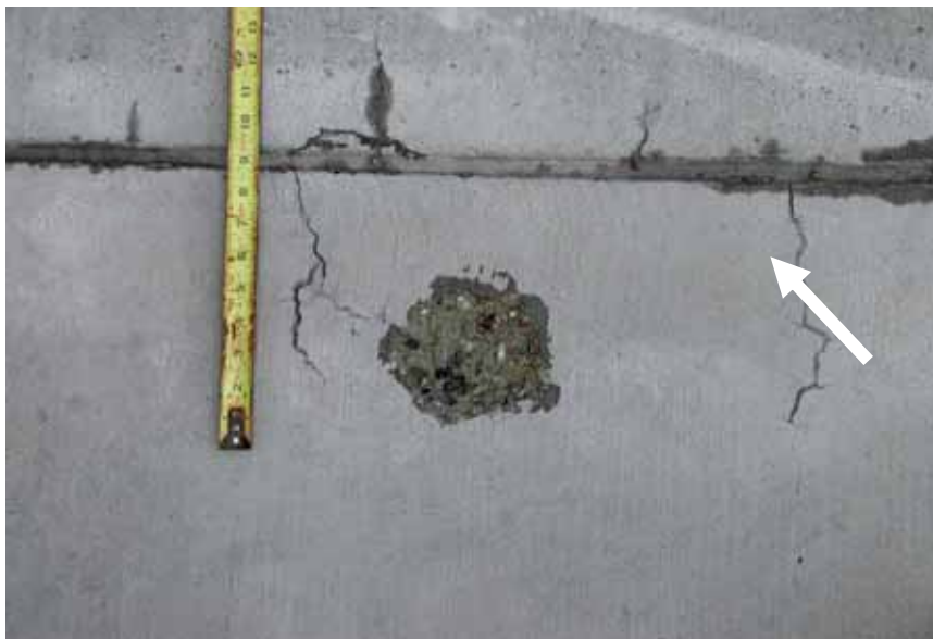
Figure 2-2. A close-up view of laddering (→).
