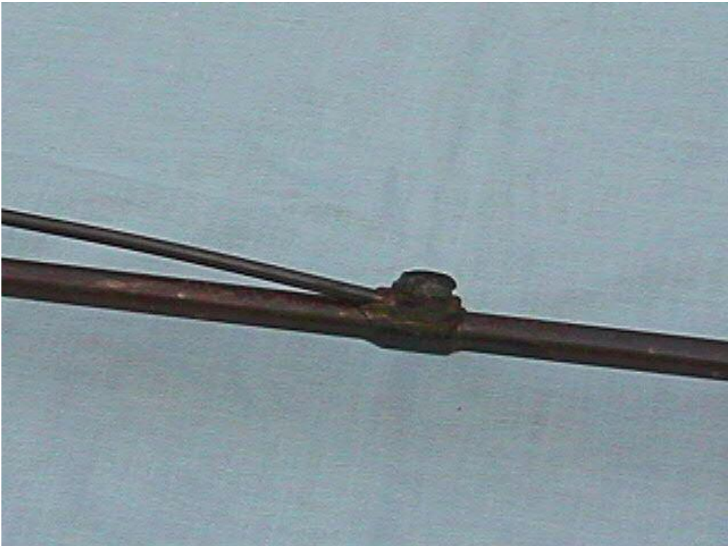
No. 3 : We can clearly see the above mentioned welding.
