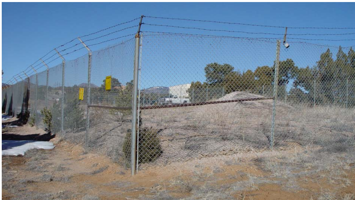
Figure 4. Material Disposal Area H at TA-54. (The mound of soil in the right forefront of the photo is clean fill remaining after the excavation of the last shaft.)
