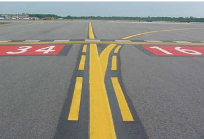
An example of the enhanced taxiway centerline paint scheme.
