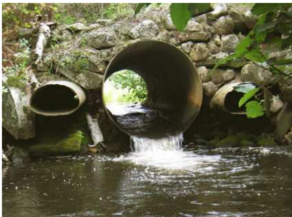
Simpson Creek culvert before project
