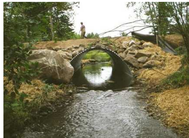
Simpson Creek culvert after project
