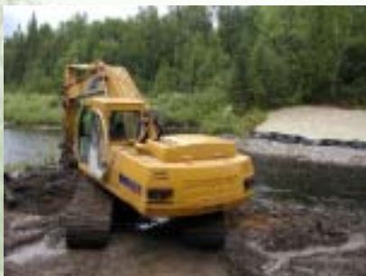
Environmentally friendly fuels were used during the dam removal process.
