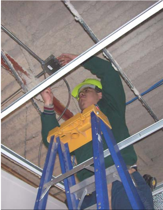
Crew Leader Arias puts the finishing touches on a junction box.
