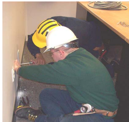
Student Foreman Seaworth assists another student in the installation of a plate cover.
