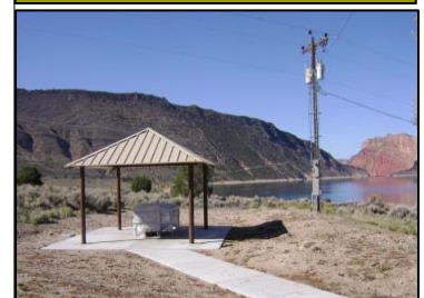
Antelope Flat: New Fish Cleaning Station
