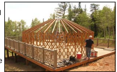
Final Stages of Yurt Rebuild Great Job YCC Crew!!!
