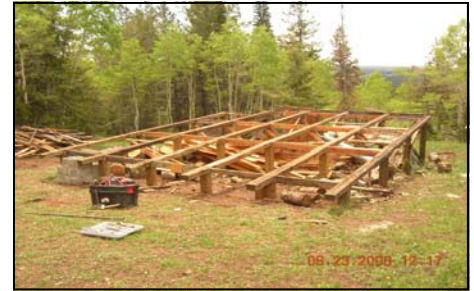
Beginning of Yurt rebuild
