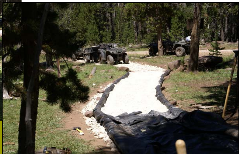
The 2008 Youth Conservation Corps Crew working to install a turnpike to improve drainage and reduce resource damage on a section of the Outlaw Trail.
