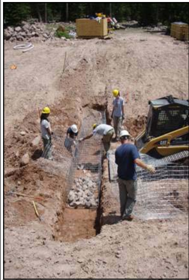
Students building gabion baskets at Brown Duck Lake
