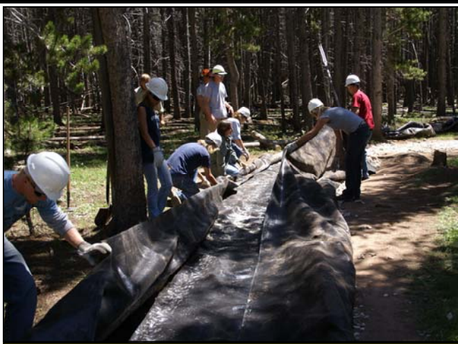
The 2008 Youth Conservation Corps Crew working to install a turnpike to improve drainage and reduce resource damage on a section of the Outlaw Trail.
