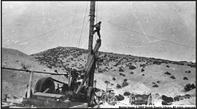
Oil well near Vernal, UT, April 26, 1913
