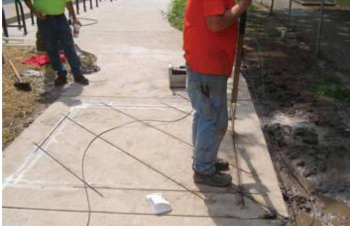
Figure 4-29. Type D loop installation (Photograph courtesy Darcy Bullock, School of Civil Engineering, Purdue University, West Lafayette, IN).
