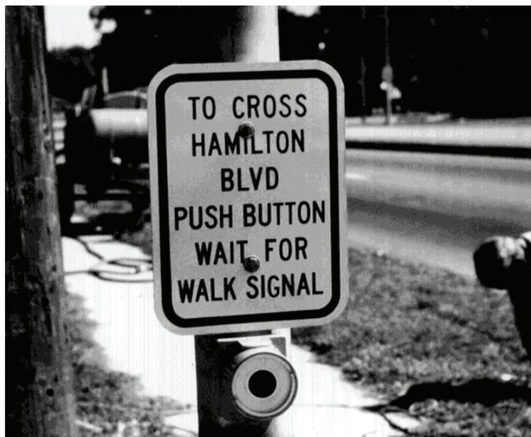
Figure 3-21. Manually operated pedestrian push button.
