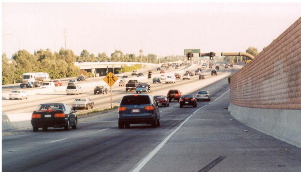
Figure 3-14. Freeway-to-freeway metering at the junction of the I-105 and I-605 freeways in Norwalk, CA (Photograph courtesy of Lawrence A. Klein).
