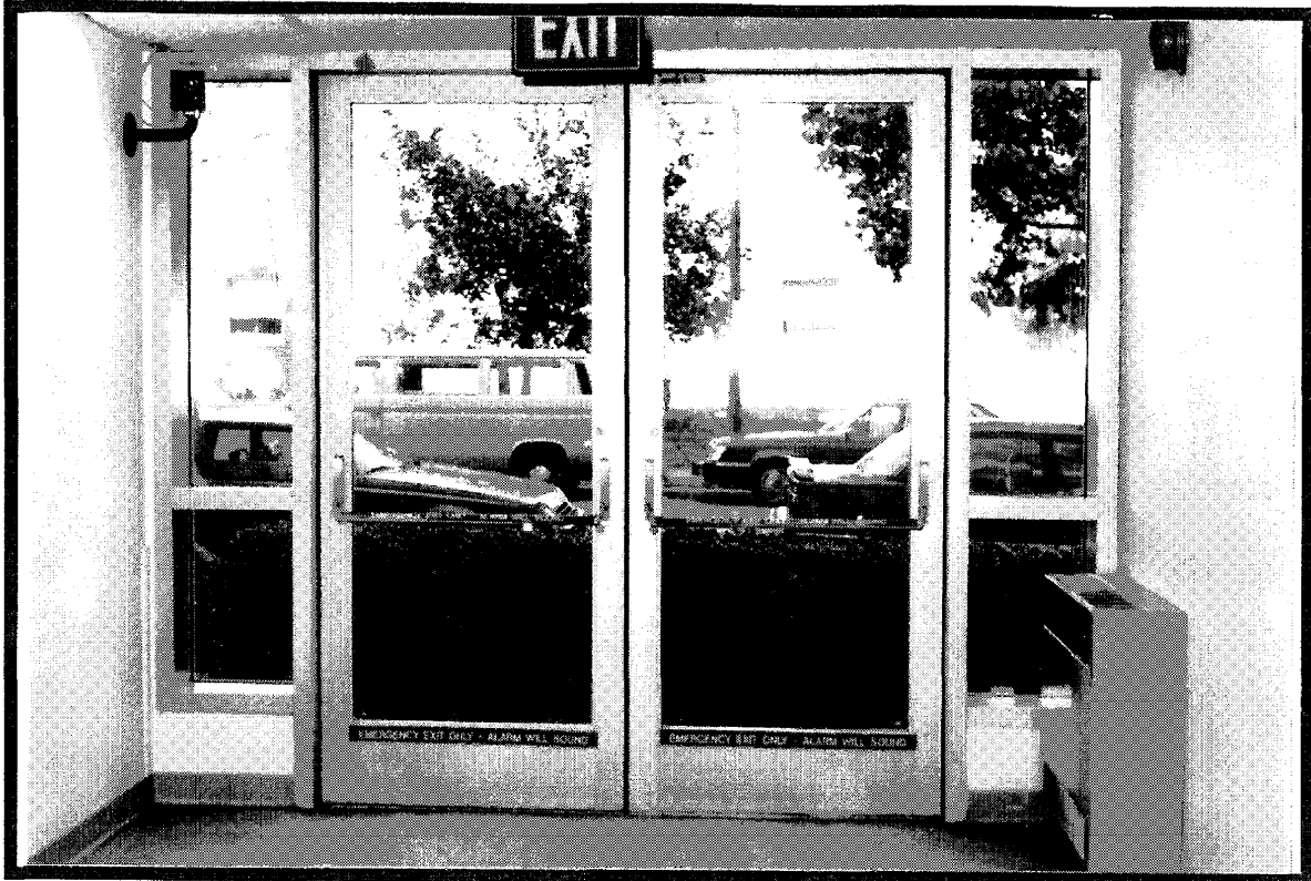
Emergency Exit - North Face - West
