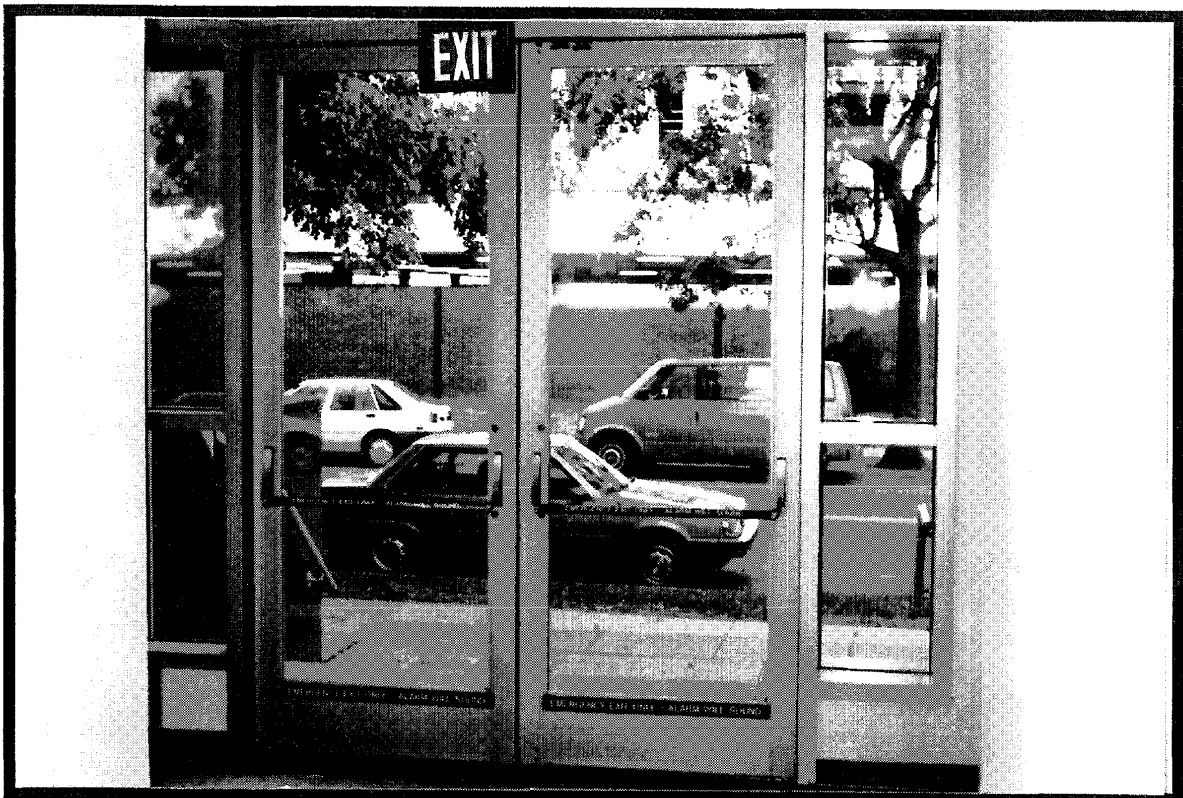
Emergency Exit - North Face - East
