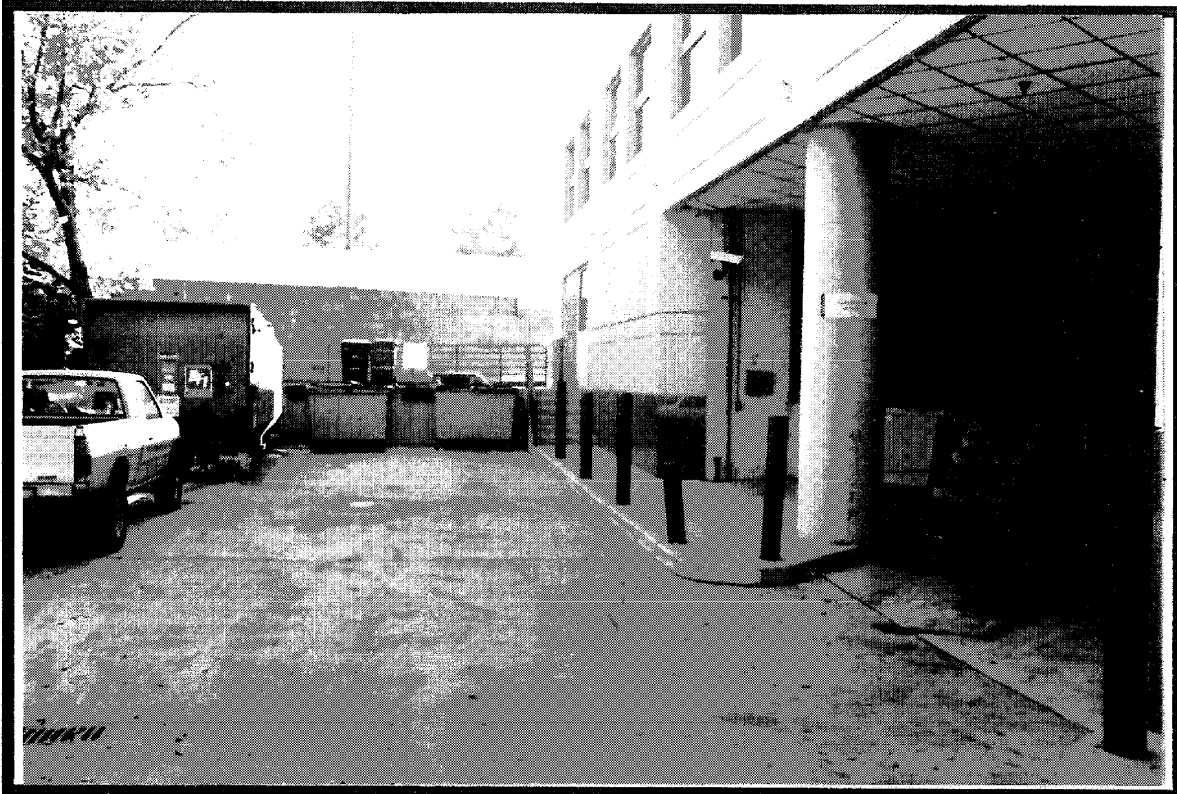
East Face - Delivery Area/Loading Dock
