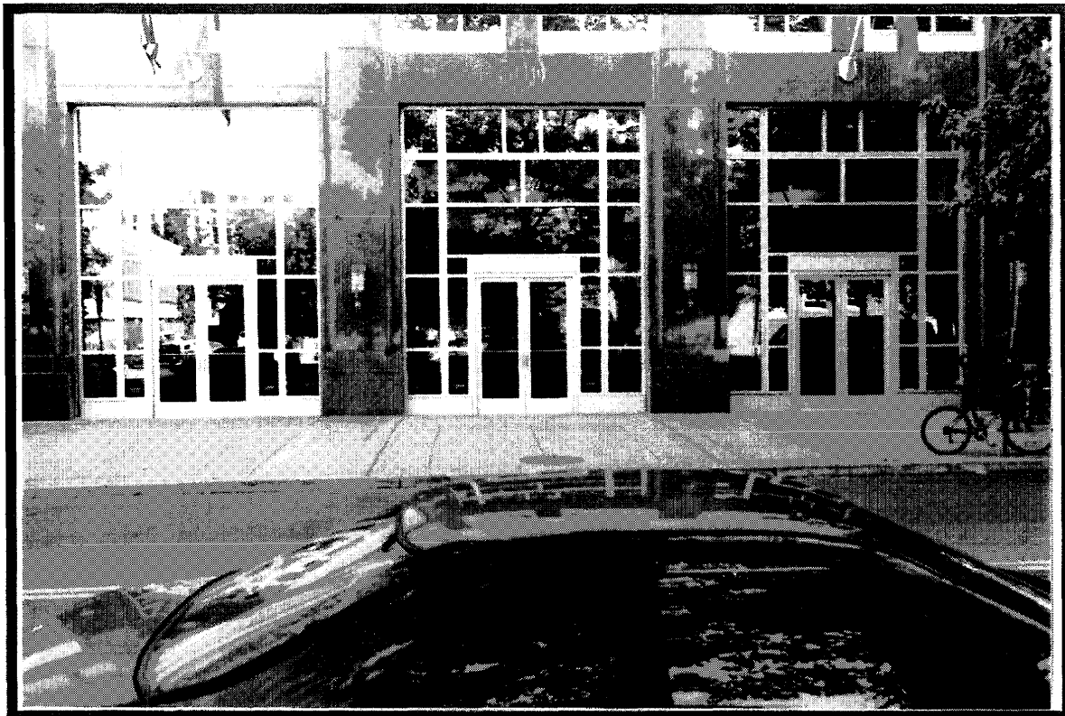
North Face – Main Entrance Doors
