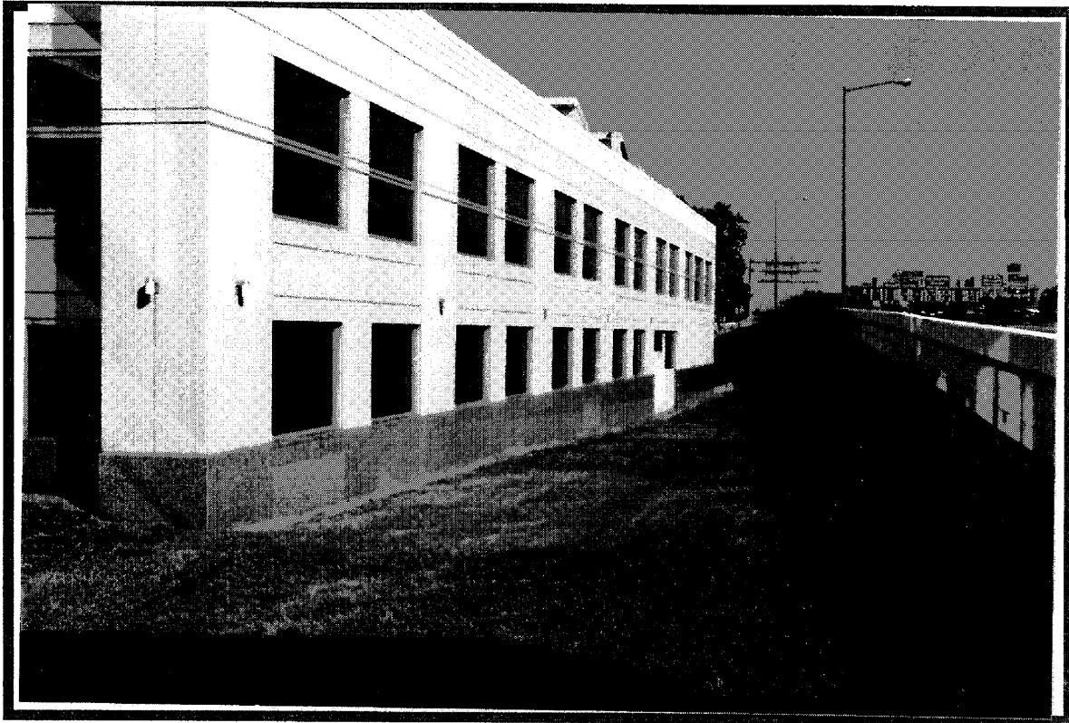
South Face – Emergency Exit
