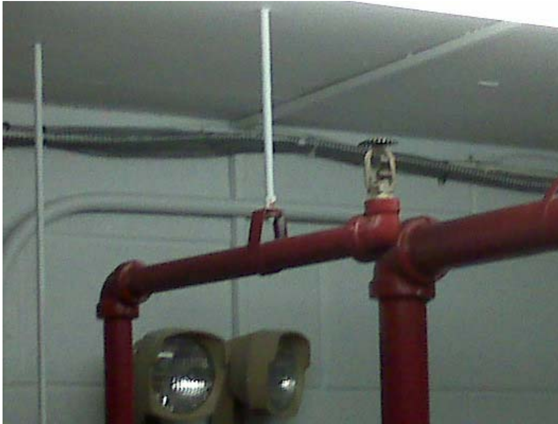
Figure I-1 Threaded rod: Use in suspending pipe
