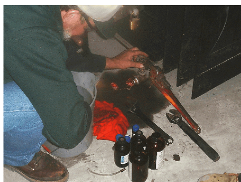
Figure 5. Flushing Sampling Port
