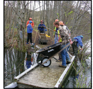
Repairing the Hummocks Trail
