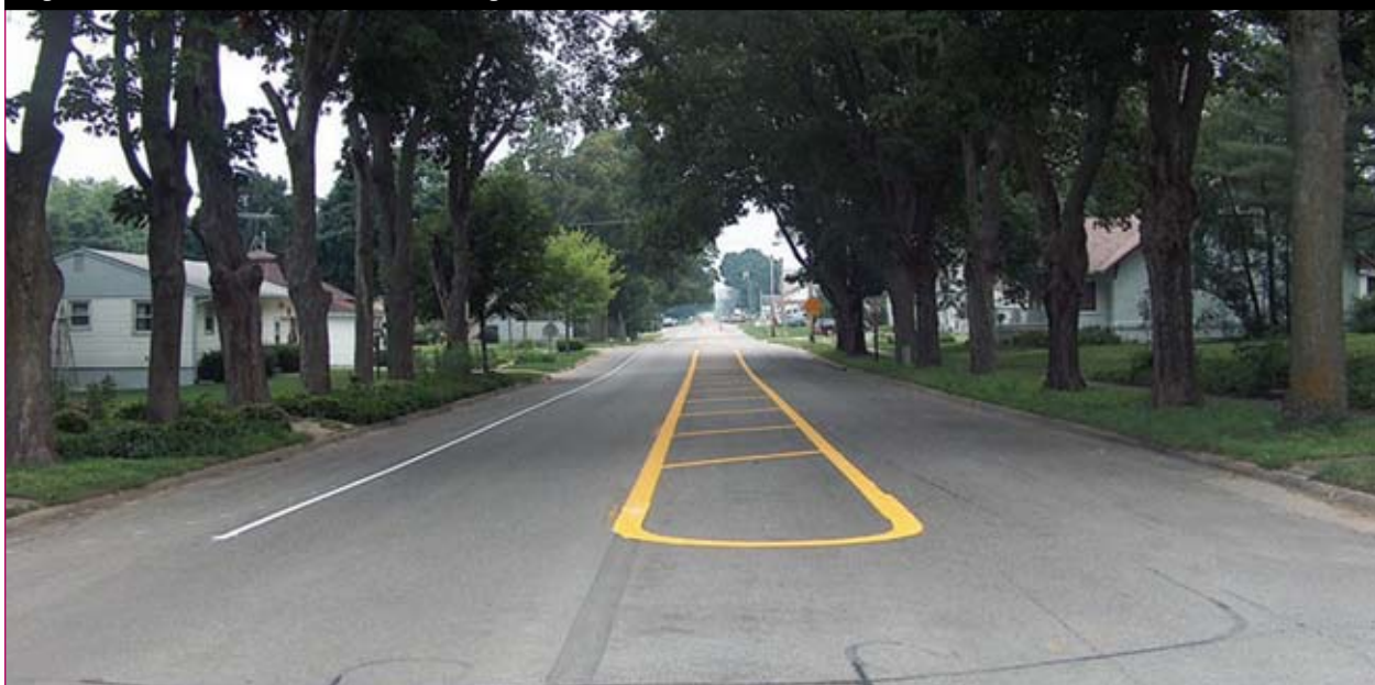
Figure 4. Painted center island and edgeline used to narrow lane.
