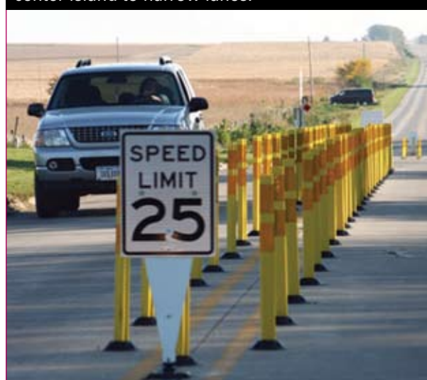
Figure 9. Tubular channelizing markers used for center island to narrow lanes.
