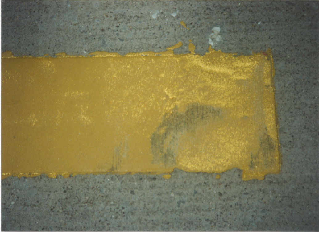
FIGURE A-20. SNOWPLOW STRIKE ON METHACRYLIC RESIN
