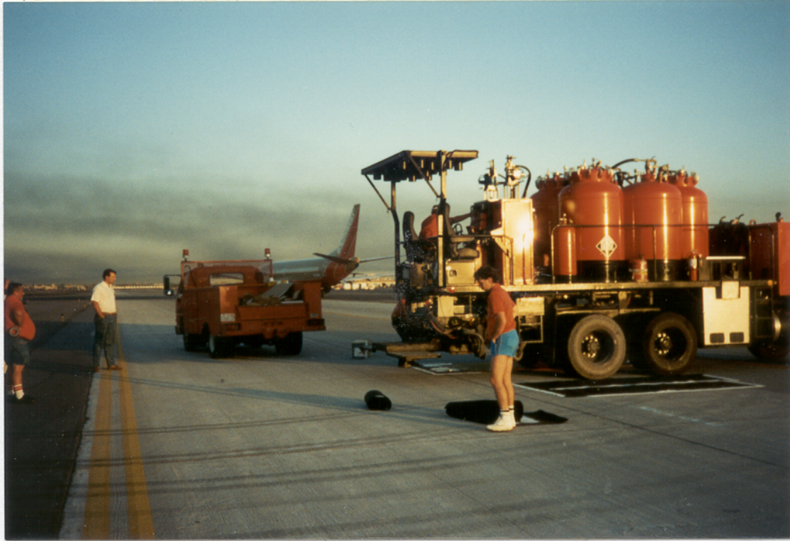
FIGURE A-12. EPOXY TEST STRIPE APPLICATION AT PHOENIX
