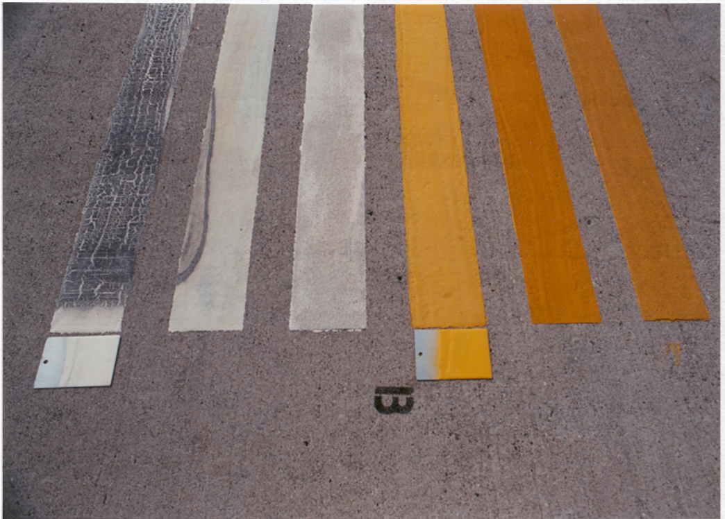
FIGURE A-21. EPOXY NO. 2 - INCOMPLETE HARDENING
