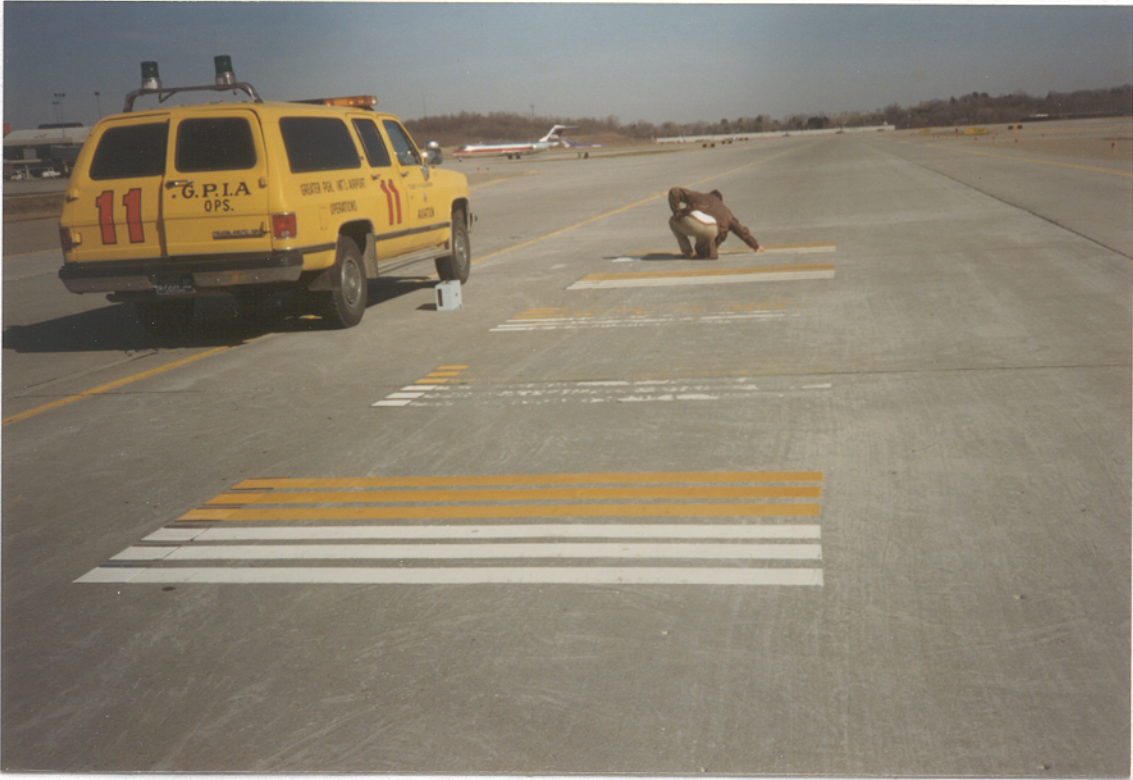
FIGURE A-26. TAXIWAY TEST STRIPES - PITTSBURGH (NORTH VIEW)
