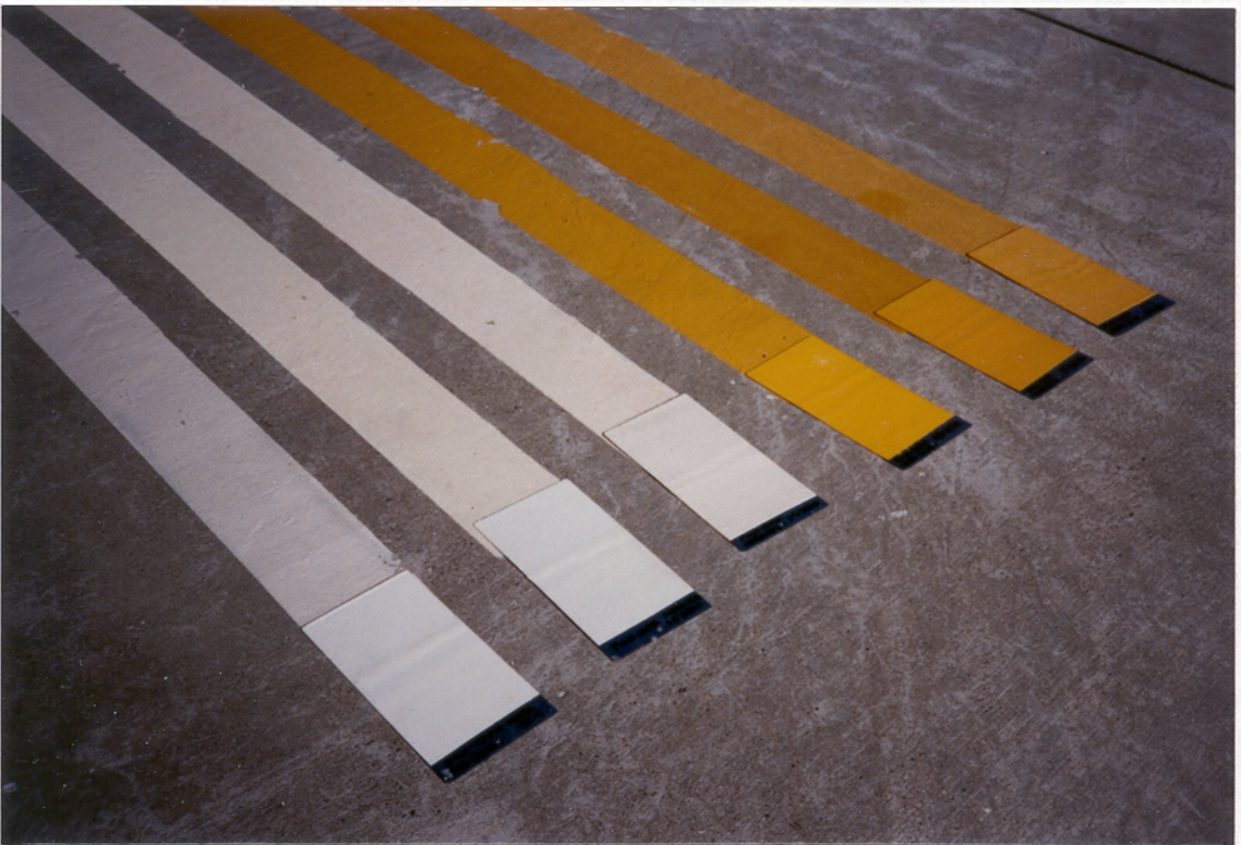
FIGURE A-29. EPOXY NO. 2 TAXIWAY TEST STRIPE AFTER 1 YEAR - PITTSBURGH
