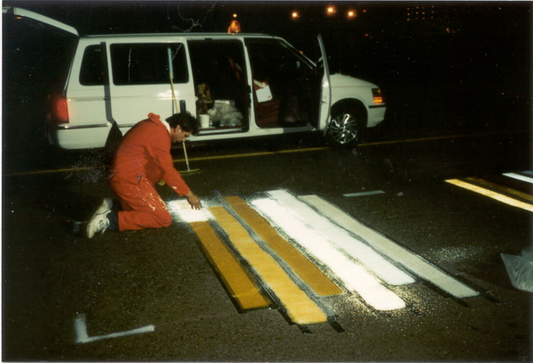
FIGURE A-10. EPOXY TAXIWAY TEST STRIPE APPLICATION
