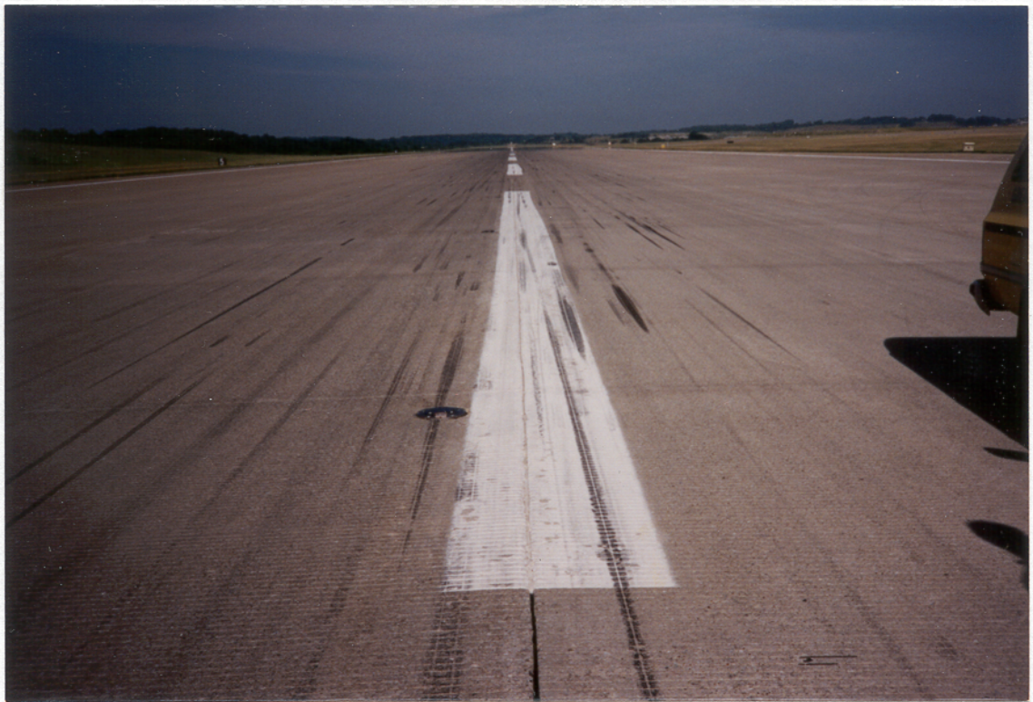
FIGURE A-33. RUNWAY TEST STRIPE AFTER 1 YEAR - PITTSBURGH
