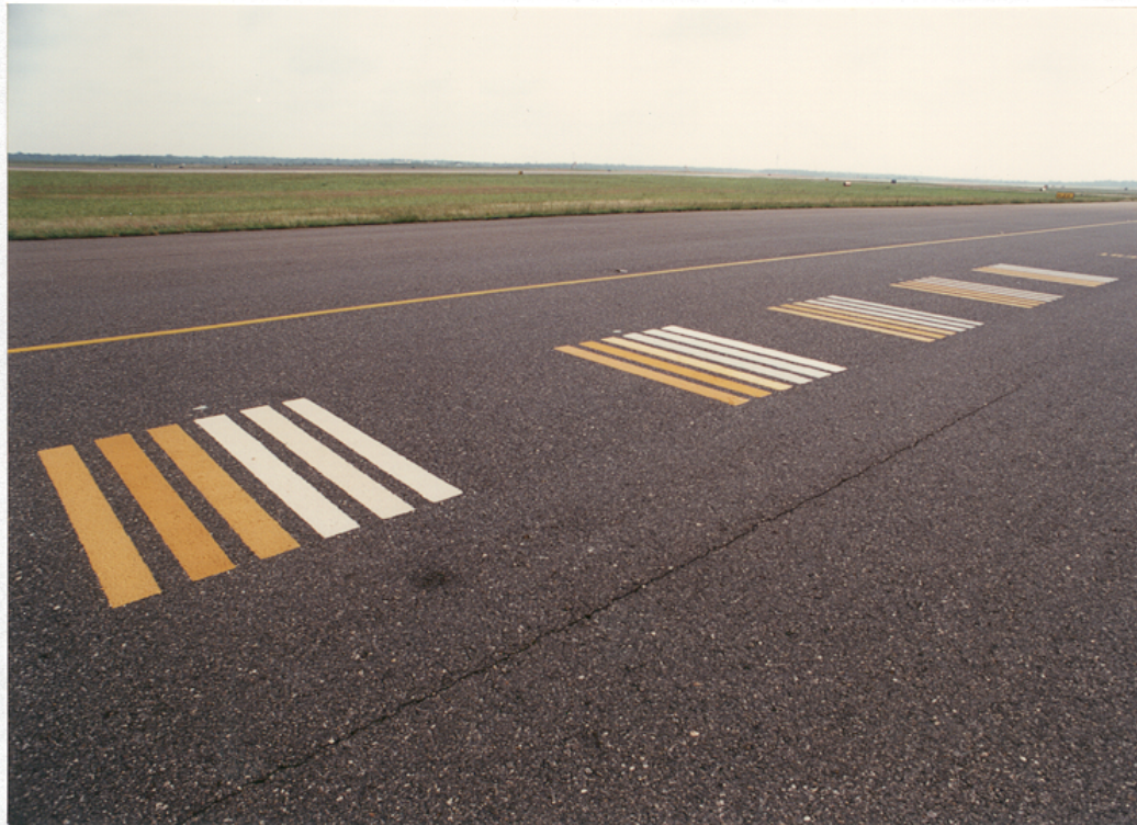
FIGURE A-15. TAXIWAY TEST STRIPES ON ASPHALT SURFACE
