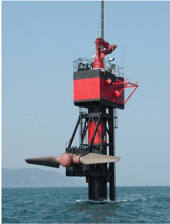
Figure 8-2 “Seaflow” device undergoing maintenance in North Devon, U.K.
