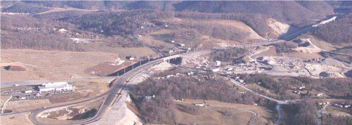
Figure 37. Photo. Aerial view of the Smart Road.
