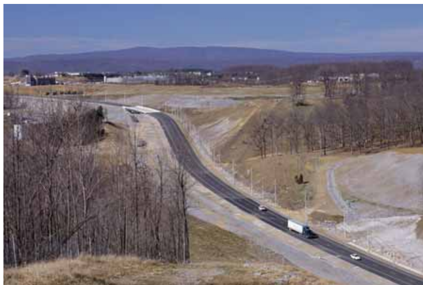
Figure 12. Photo. Smart Road.
