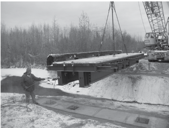
An Alaska General Contractors' construction crew eases Airway Drive bridge into place.
