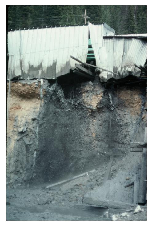
**Figure 29.** Erosion trench and muddy discharge at American tunnel portal, June 5, 1978, the day after Lake Emma flood. With 2,000 ft of head pressure, Lake Emma water exited the American tunnel (mine # 96) like a huge fire hose, blowing open the building wall and eroding the dump back about 15 ft, creating an erosion trench. The scene was described by witnesses as something out of a science fiction movie.
