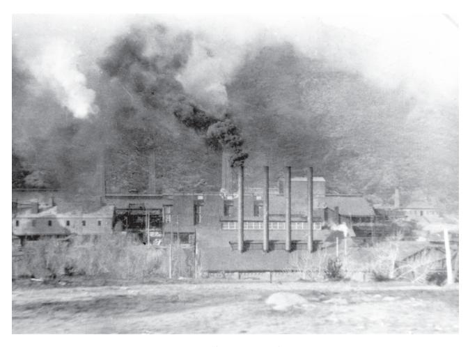
**Figure 6.** Durango Smelter along the Animas River, 1906 (C.A. Chase photo). Silverton lead-silver ores were shipped to the smelter in Durango for processing into metal. The process produced considerable air pollution.
