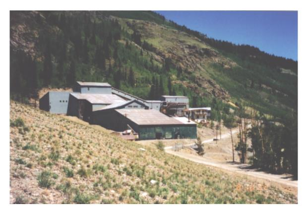
**Figure 20.** Mayflower Mill (site # 221) and reclaimed tailings (sites # 507–510, fig. 2; 2002). Also known as the Shenandoah-Dives Mill, it operated for over 60 years (1930–1991). The aerial tram (AA, fig. 2) entered the plant at far right while tailings were stacked in tailings ponds on the left (# 507–510). These tailings were capped and seeded during 1990s reclamation work by Sunnyside Gold Corp. In 2001 the mill was designated a National Historic Landmark by the Secretary of the Interior.
