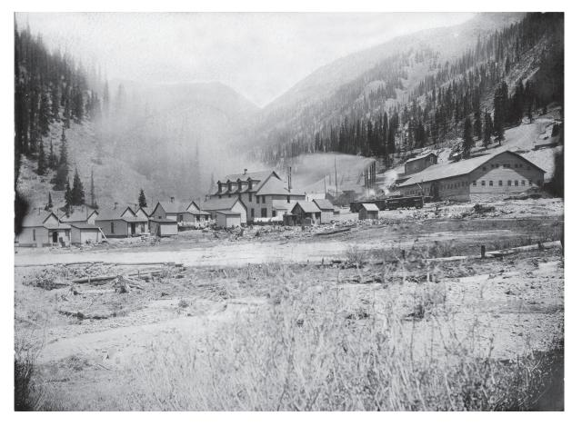
**Figure 14.** Gold King Mill (site # 94, fig. 2) at Gladstone and SG&N Railroad (circa 1903). Tailings from the Gold King Mill can be seen crudely impounded by log dams along Cement Creek. The aerial tram (D, fig. 2) entered the building from the upper right; boxcars for concentrate shipment waited along the railroad sidings.
