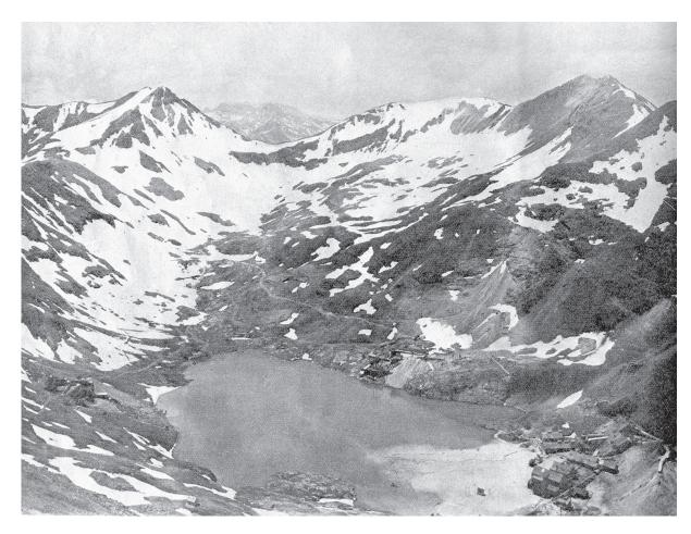
Figure 13. Silver Lake (mine # 343) and adjacent mines, mill, and mill tailings (Silverton Miner, 1907). The Silver Lake Mill # 1 (site # 347, fig. 2) at lower right was the first successful low-grade concentrator in the area. Tailings slowly filled the north end of the lake but were later removed. See also figures 15 and 16. The lowa (mine # 345) is in center on right side of lake; Royal Tiger (mine # 348) is on left side of lake.
