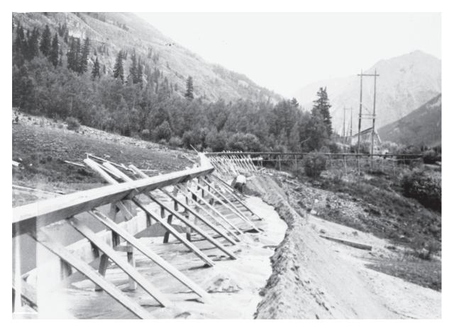
**Figure 24.** Mill tailings spigots at tailings pond #1, Mayflower Mill (site #221, circa 1934; C.A. Chase photo). Wooden flumes were used to slurry tailings for disposal into tailings ponds (#507, fig. 2) rather than into the river. Holes in the bottom of the flume let coarser sands flow down the planks into piles, which were shoveled together to create the pond wall while water settled behind the resulting dam.
