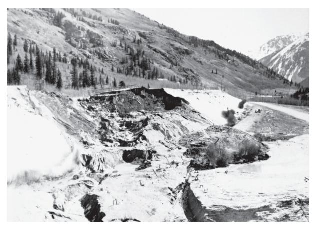
**Figure 26.** Failure of tailings pond # 1 sand wall dam (site # 507) at Mayflower Mill (1947; C.A. Chase photo). As sand walls became higher, structural instabilities also increased. Ice lenses in the wall were partly to blame for this 1947 collapse. The 1974 wall failure would be just out of this view to the left. Reclaimed tailings are shown in figure 20 to left of Mayflower Mill.
