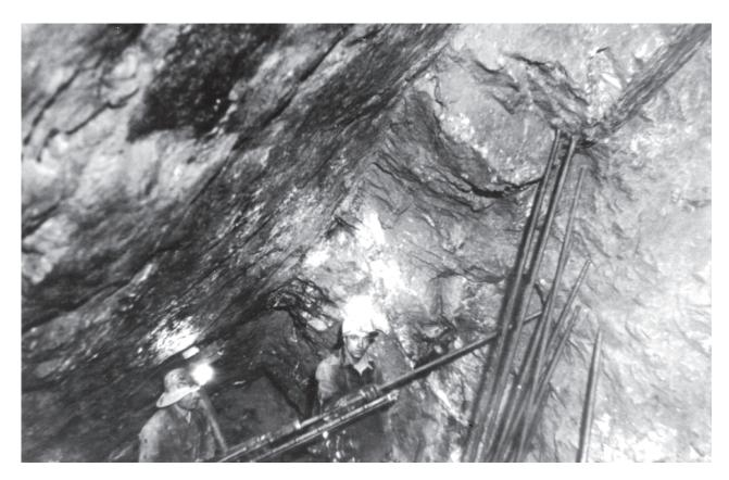
**Figure 17.** Shrink stope mining in Shenandoah-Dives (mine # 355, 1937; C.A. Chase photo). Air drills increased productivity and size of the mines. Here a Leyner type drill is working a flat-lying stope. In the shrinkage method, the miners stand on the ore pile which is later completely removed for processing, leaving a void. Vein exposed is about 3 ft thick.
