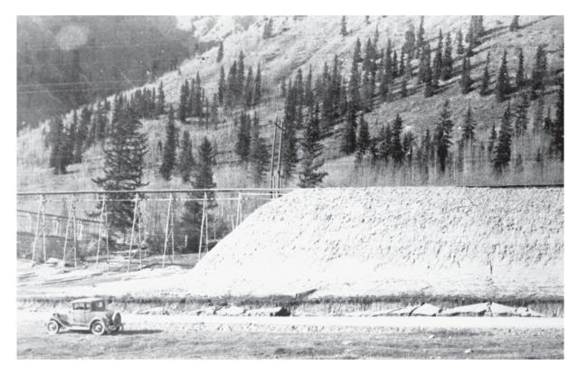
**Figure 25.** Tailings pond # 1 sand wall (site # 507) at Mayflower Mill (1936; C.A. Chase photo). As tailings were deposited the sand walls became higher. Tall flumes (shown on left of sand wall) called "launders" now were needed to transport the sand and water.
