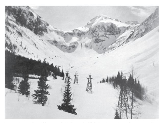
Figure 8. Iowa aerial tram (Y, fig. 2 and table 3) in Arrastra Creek (C.A. Chase Photo 1925). Aerial tramways provided the key link between high-altitude mines and the mills and railroads located along the river. The lowa tram is nearly 3 miles long and climbed the steep cliff to Arrastra Basin in the background. The Silver Lake tram is out of sight in the trees to the left.
