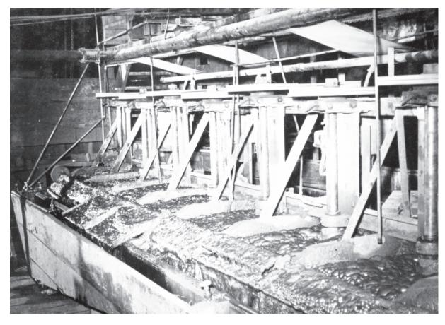
**Figure 18.** Minerals Separation flotation cells, Mayflower Mill, 1930 (site # 221, fig. 2; C.A. Chase photo). The flotation process created froth, which floated the ore particles out of the redwood cells or tanks. The Minerals Separation Syndicate was the leading patent holder in the early years.
