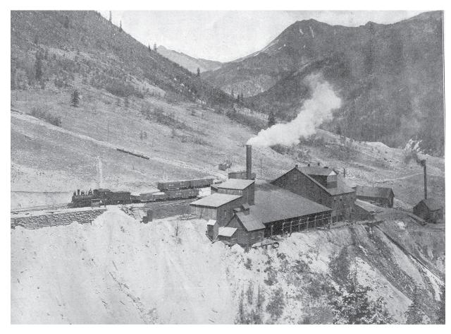
**Figure 7.** Kendrick-Gelder (aka Ross) Smelter (site # 213, fig. 2) in Silverton and SG&N Railroad (circa 1907). Silverton had several short-lived smelters, connected to the mines by the narrow gauge railroad system. These small plants were uneconomic except during periods of high metal prices.
