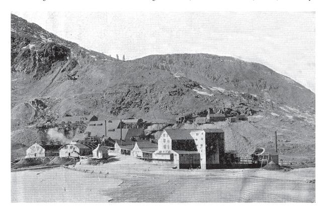
**Figure 15.** Silver Lake Mill # 1 (site # 347, fig. 2) discharging tailings into Silver Lake (Silverton Standard folio, 1904). The tailing flume from the mill is discharging tailings onto the sand pile now filling Silver Lake (see fig. 13). The large building is the miners' bunkhouse.
