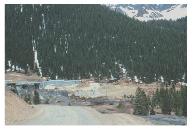
**Figure 28.** American tunnel portal (mine # 96) June 5, 1978, the day after the Lake Emma flood. Lake Emma water and mud discharged at the American tunnel portal at Gladstone some 2,000 ft below and 2 miles away from Lake Emma. Black mud was deposited over the dumps and into Cement Creek. Portal buildings are on the site of the Gold King Mill (site # 94, fig. 2). Only one small house remains of the town of Gladstone circa 1903 (fig. 14). Photo taken 22 hours after the event.
