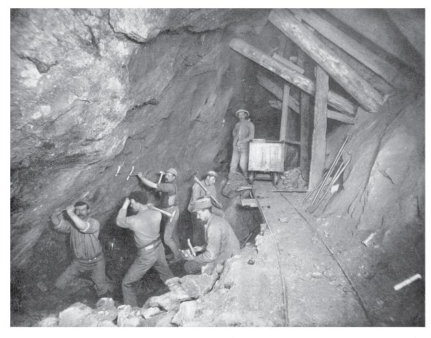
**Figure 5.** Miners working inside a cut-and-fill stope, Gold King (mine # 111; circa 1899, Silverton Standard folio, 1904). This rare view inside a stope was staged for promotional purposes, but the photo shows hand drilling on a stope hanging wall and ore being cobbed with a hammer while an engineer studies samples. Miners are working off a fill pile while timbers support mined-out area above.
