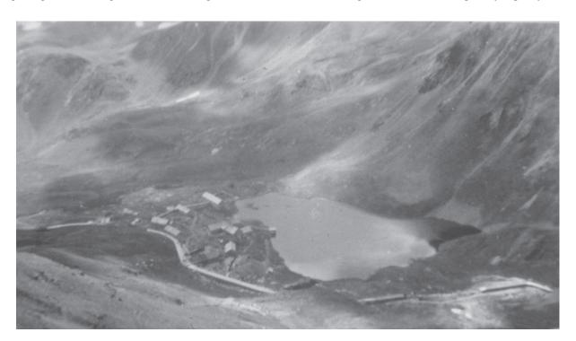
**Figure 23.** Lake Emma and Sunnyside mine from Hanson Peak (circa 1940; H.H. Mellus photo, SJCHS collection). The original Sunnyside mine (mine # 116, fig. 1) was located at 12,300 ft on the shore of Lake Emma, which was dammed to provide water to mills downstream. Men lived in the building complex; snow sheds connected them to the tunnels and shafts.
