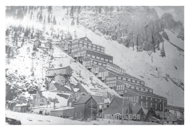
Figure 19. New Sunnyside Eureka Flotation Mill (site # 164, fig. 2), a large flotation mill built at Eureka, Colo. (circa 1925, SJCHS collection). The new 600 ton/day (later 1,000 ton/day) Sunnyside Eureka Mill dwarfs the original 150 ton/day concentrator (Sunnyside Mill # 2, site # 165, fig. 2) built in 1899, graphically showing the dramatic increase in size and scope of later milling operations.
