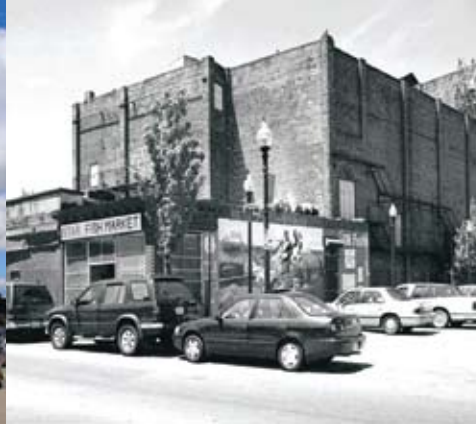
Before redevelopment, the Beethoven Theater sat vacant for more than 30 years.
