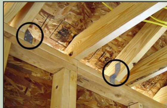
Above: Hurricane clips attaching roof trusses to side walls.
