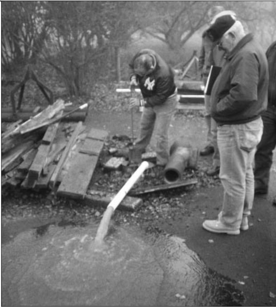
The small system operator shown above is flushing iron from the water system's distribution system. More than 3,100 small systems have an unmet need to treat for iron and manganese. These secondary contaminants make water reddish-brown and stain sinks and laundry.
