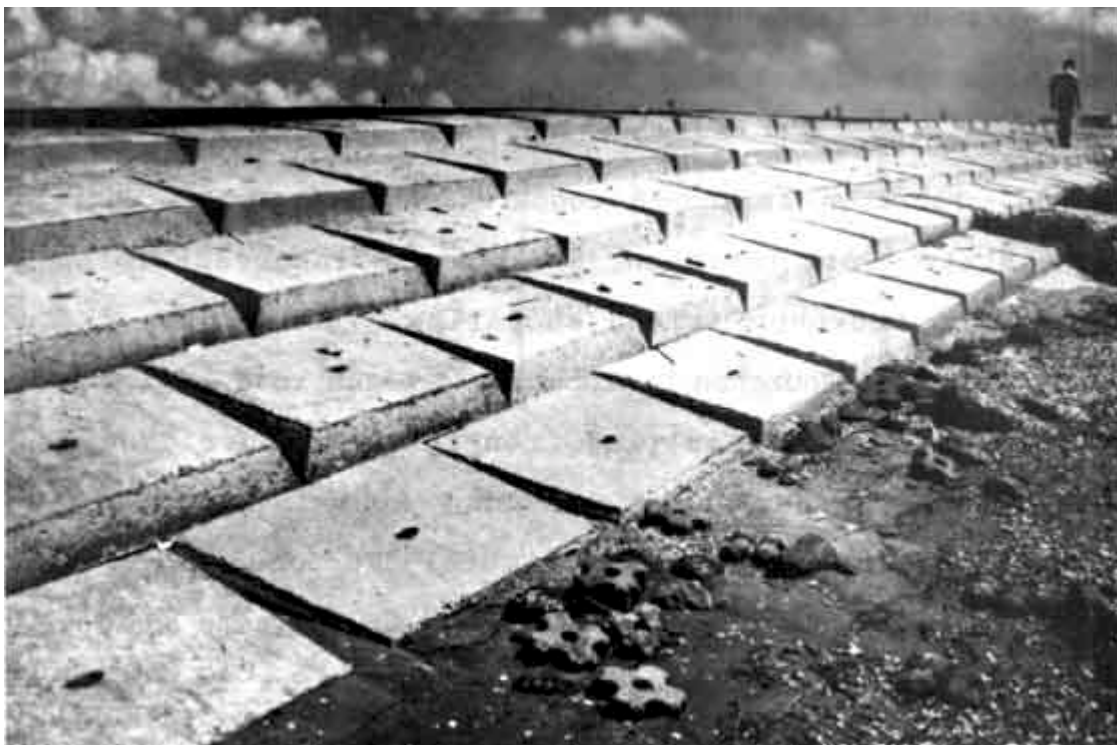
Figure 24. New revetment installed to protect the shoreline and Highway 82 in Cameron Parish, LA.
