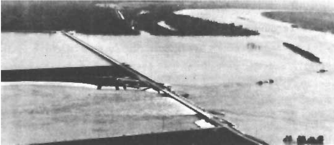
Figure 7. Old River Control Structure near Simmesport, Louisiana.
