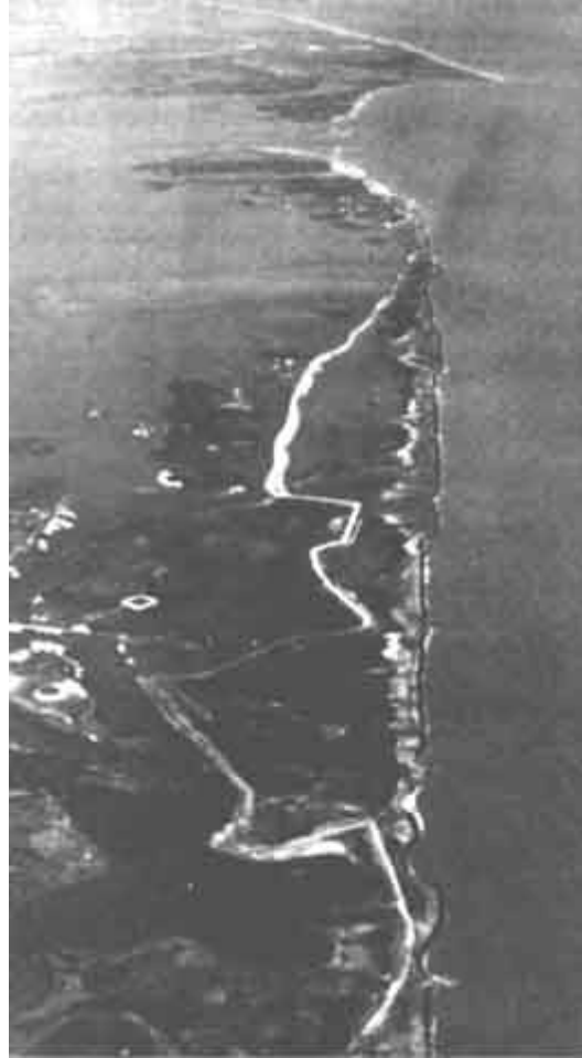
Figure 29. East Timbalier Island. Note that the island has continued to subside and wash away despite all company efforts to encircle the island with rock sea walls.
