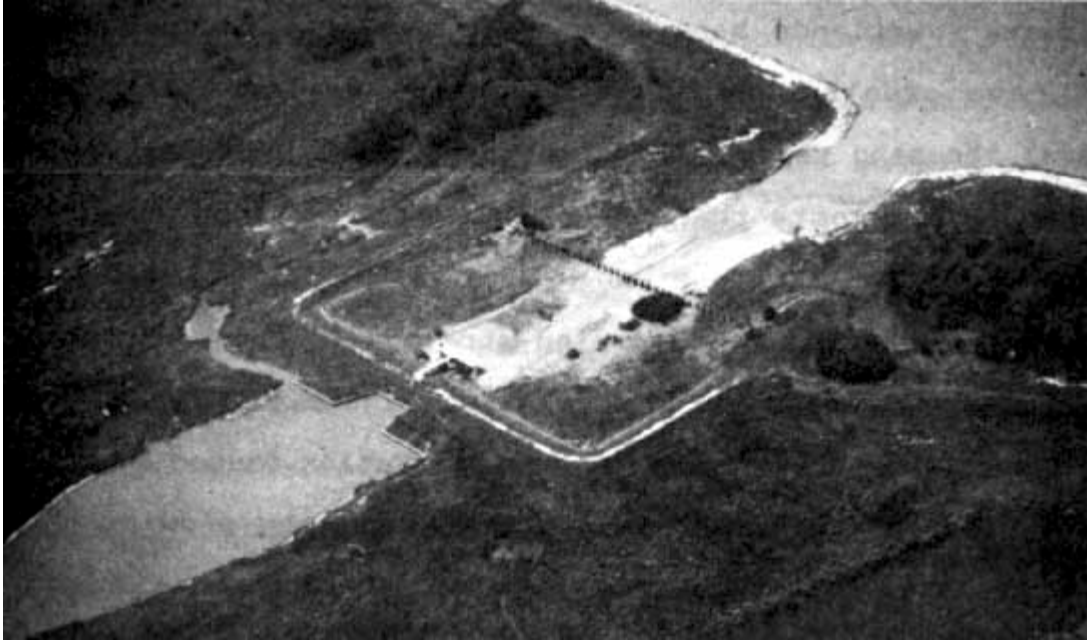
Figure 21. Freshwater diversion structure at Bayou LaMoque in Plaquemines Parish, LA.
