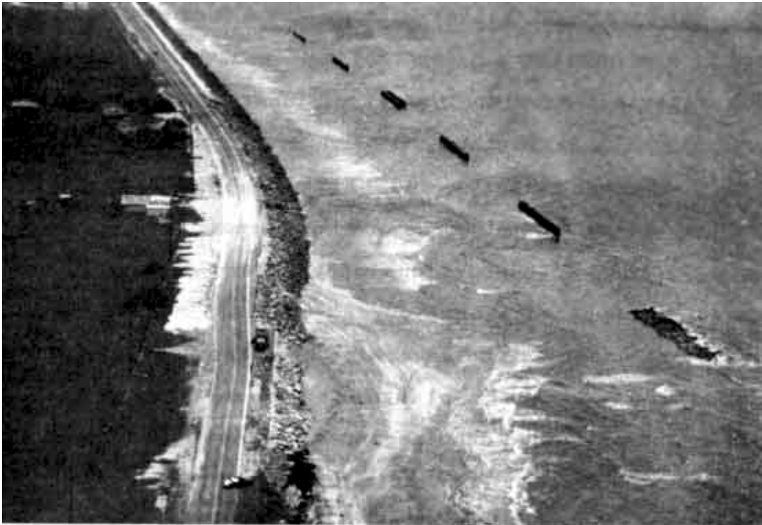
Figure 25. Six experimental breakwaters constructed west of Holly Beach, LA. To help protect Highway 82 from storm impacts.
