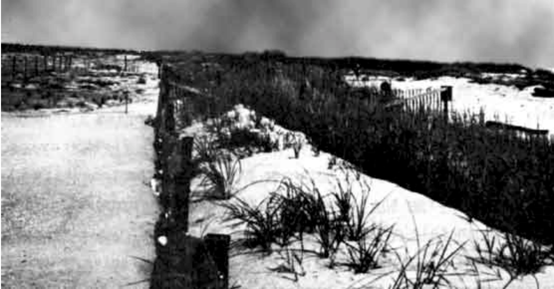
Figure 30. Sand fencing and vegetation plantings help build and stabilize barrier island sand dunes.
