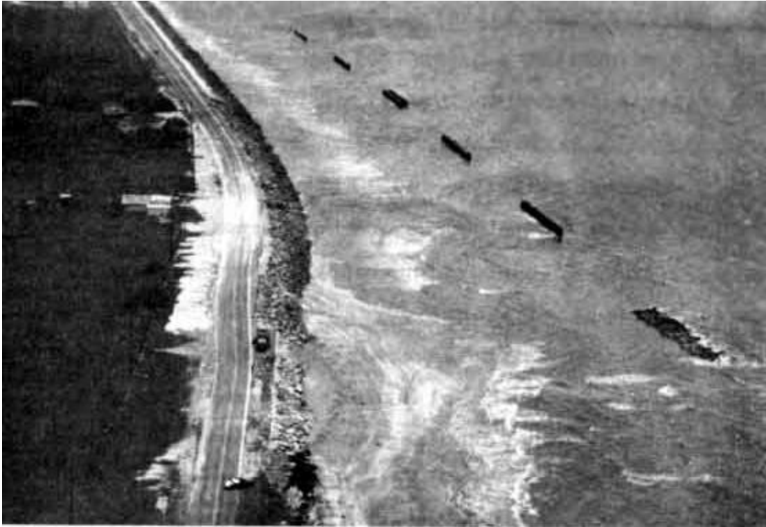
Figure 25. Six experimental breakwaters constructed west of Holly Beach, LA. To help protect Highway 82 from storm impacts.
