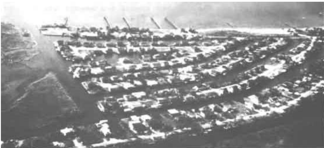
Figure 9. Wetlands dredged and filled for residential development along the north shore of Lake Pontchartrain.
