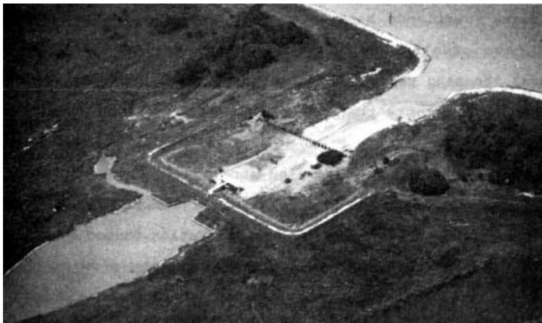
Figure 21. Freshwater diversion structure at Bayou LaMoque in Plaquemines Parish, LA.
