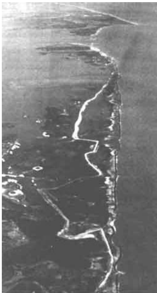
Figure 29. East Timbalier Island. Note that the island has continued to subside and wash away despite all company efforts to encircle the island with rock sea walls.
