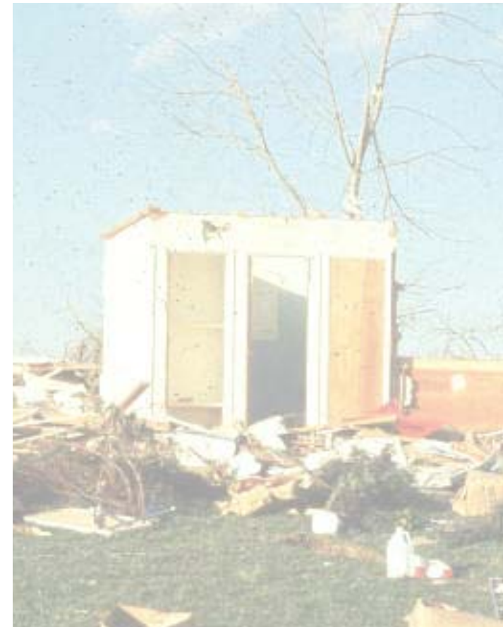
An F2 tornado struck New Hope (Madison Co. AL) on November 24, 2001. This storm shelter remained completely intact while the house nearby was destroyed.
