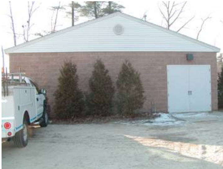
Water Treatment Building For Windham Public Water Windham, NH
