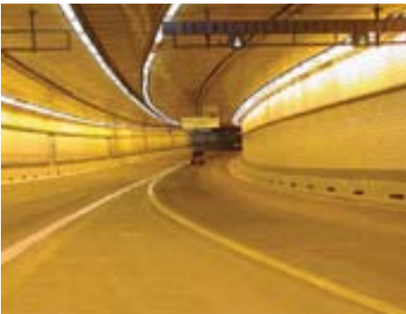
Ted Williams Tunnel
