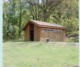
Outdated vault toilets have been replaced by new flush toilets.
