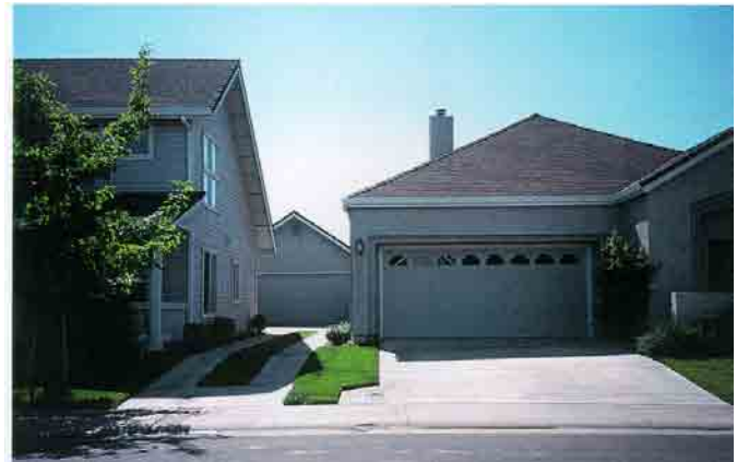
DESIRABLE SIDEDRIVE W/ REAR GARAGE
