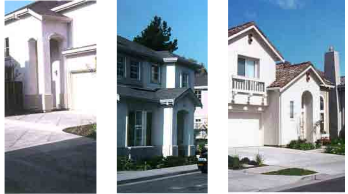
Undesirable Entries: Entries are frequently minimal and the homes lack the transition space between the street and living spaces as well as the architectural detail which porches can provide.
