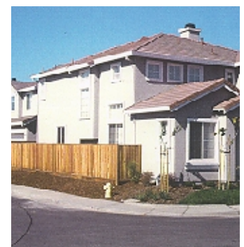
Undesirable: Buildings with blank facades, lacking architectural detail and blank side-yard fencing.
